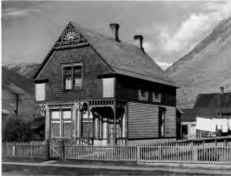
This house in Silverton Historic District NHL displays the pride of its builder despite the town's isolation. Photo by Russell Lee. Reproduced from the collection of the Library of Congress.
