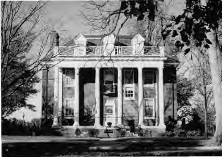
Quarters 7 at Fort McNair in Washington DC. This quarters, designed by McKim, Meade and White, is representative of 15 similar General's Quarters in a row. Photo by Nat McCormick.
