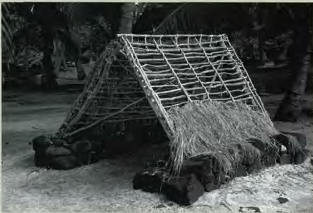
Reconstruction of a hale pili used for storage on the royal palace grounds at Hōnaunau. Photo by Bill Chapman.
