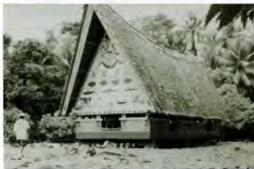
A bai, a traditional men's meeting house, which was built three years ago on a traditional bai platform in the state of Airai, Palau. Photo by Kimberlee Kihleng.
