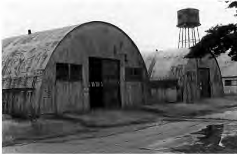
Two of the 17 Quonsets at Camp Endicott in Davisville, Rhode Island, that were listed in the National Register of Historic Places for their architectural, engineering, and military significance in 1977, more than a decade before they reached their 50th anniversary. Photo by the author.
