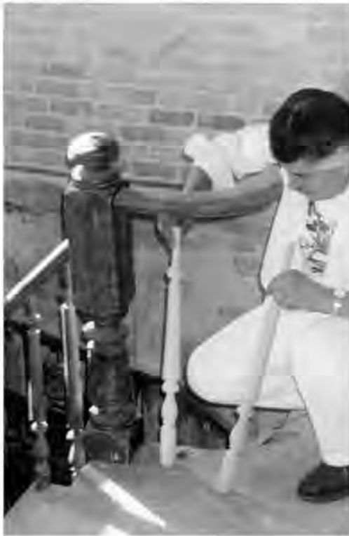
Donn Brunson, historical restoration instructor and avid paint specialist, positions new wood turns in the staircase of the historic Band Building. The replacements, made of hemlock, are authentic reproductions of the original.
