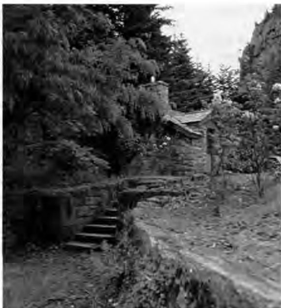
Administrative headquarters, Beacon Rock State Park. Photo by Matt Meacham, 1995.
