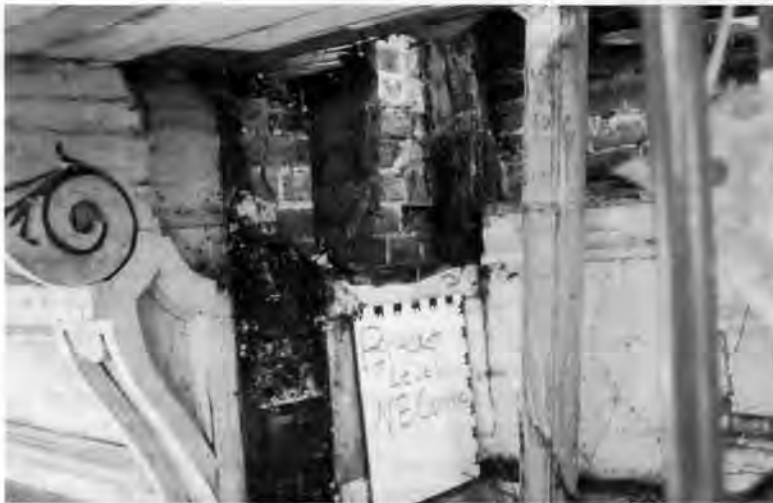
Tower bracket before restoration. Below: Same corner with new bracket trim.
