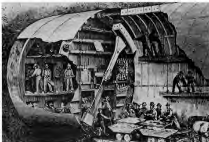
Excavating and assembling the cast iron tunnel lining. Scientific American , August 9, 1890.
