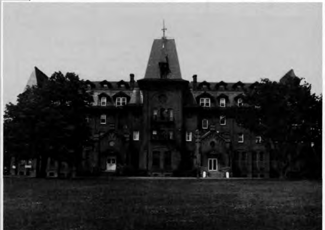
Virginia Hall (west elevation), Hampton University, Hampton, VA, 1988.
