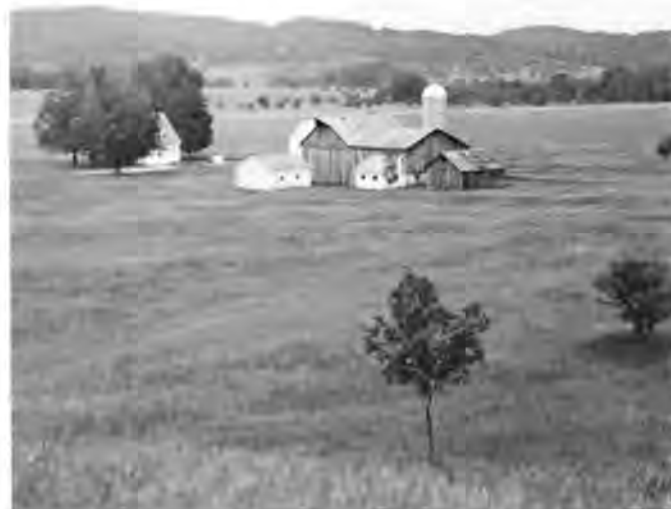
View of the Klett Farm and surrounding landscape, Sleeping Bear Dunes National Lakeshore, Michigan, 1990. Photo: John McWilliams, Historic American Buildings Survey (HABS)
