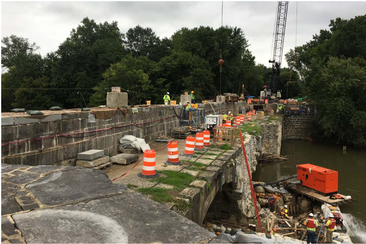
Construction work on Conococheague Aqueduct. Photo by Joe Reed.
