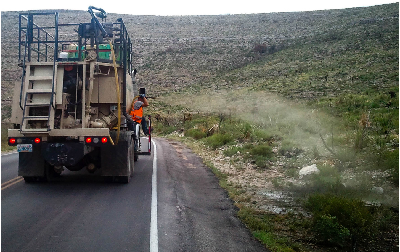
Hydro-seeding with native plant seed mix along Walnut Canyon Road, August 2012. This treatment helped revegetate several sites that had been burned through by the Loop Fire of 2011. NPS Photo.
