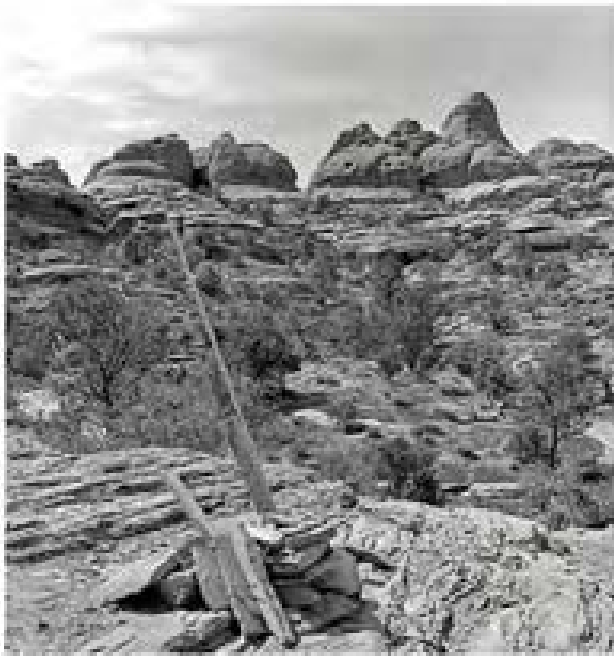
Figure 69: Road survey marker at Big Spring Canyon. C36552.592, SEUG Photographic Archives. This wood and rock cairn was located where the bridge was to cross Big Spring Canyon.
