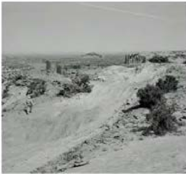
Figure 51: Road construction, The Neck, 1960s. C 40911.103, SEUG Photographic Archives.
