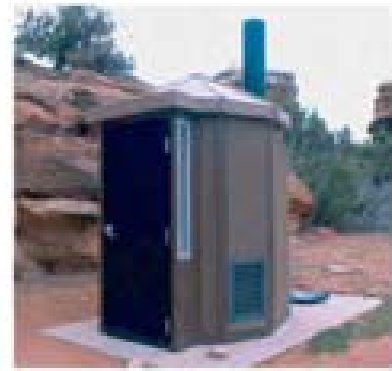
Vault toilet, Needles District. Photograph by the author.
