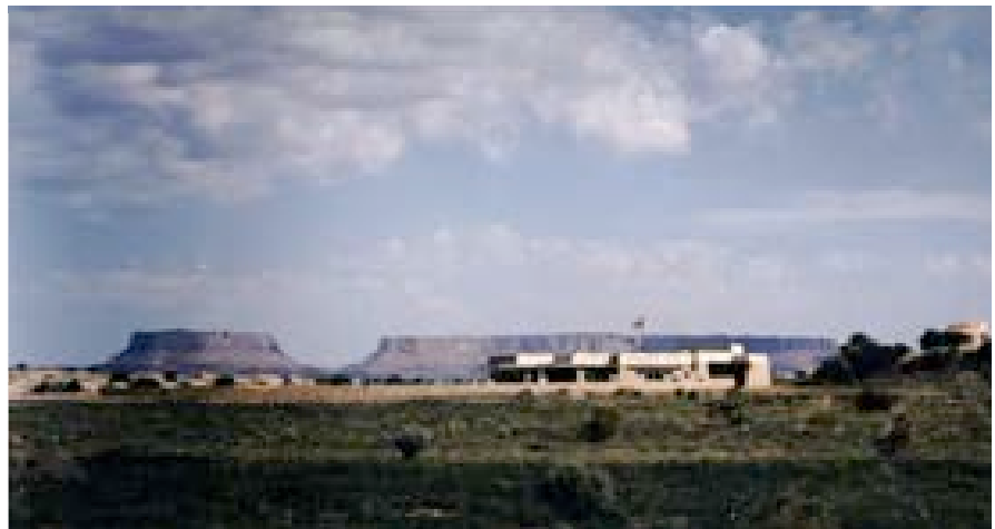
Figure 96: Completed Needles District Visitor Center. C 36299, SEUG Photographic Archives.
