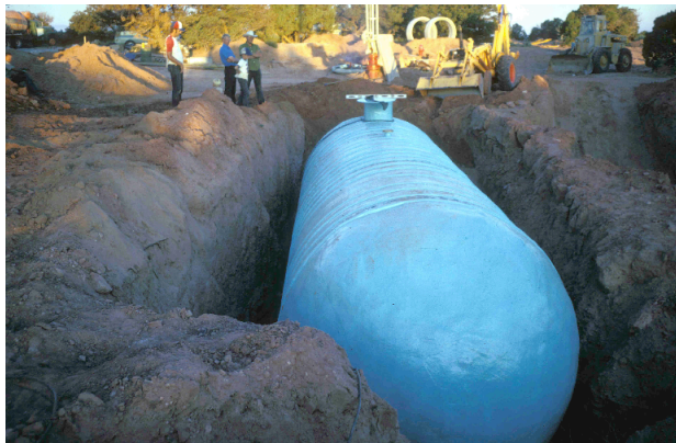
Water tank installation
