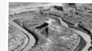
TURKS HEAD is a small tower inside a bend of the Green River.
