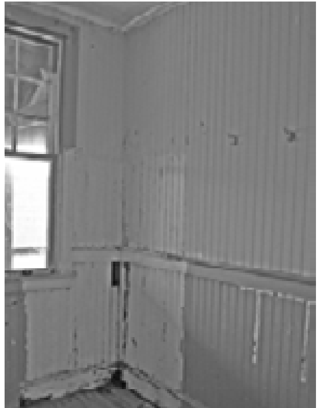
FIGURE 95. View west in Room 101. (T. Jones, NPS, 2005)
