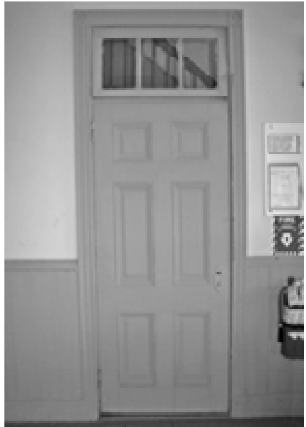
FIGURE 110. View of door in Room 104. (T. Jones, NPS, 2005)
