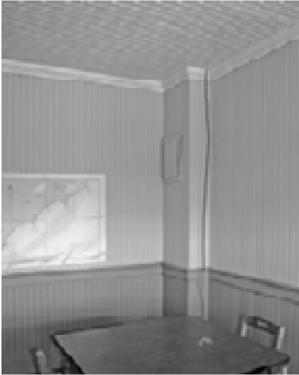
FIGURE 97. View east in Room 102. (T. Jones, NPS, 2005)
