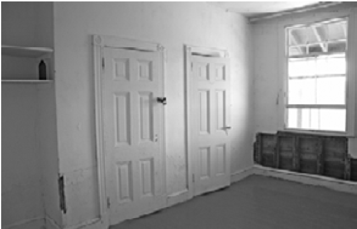
FIGURE 117. View west in Room 106. (T. Jones, NPS, 2005)
