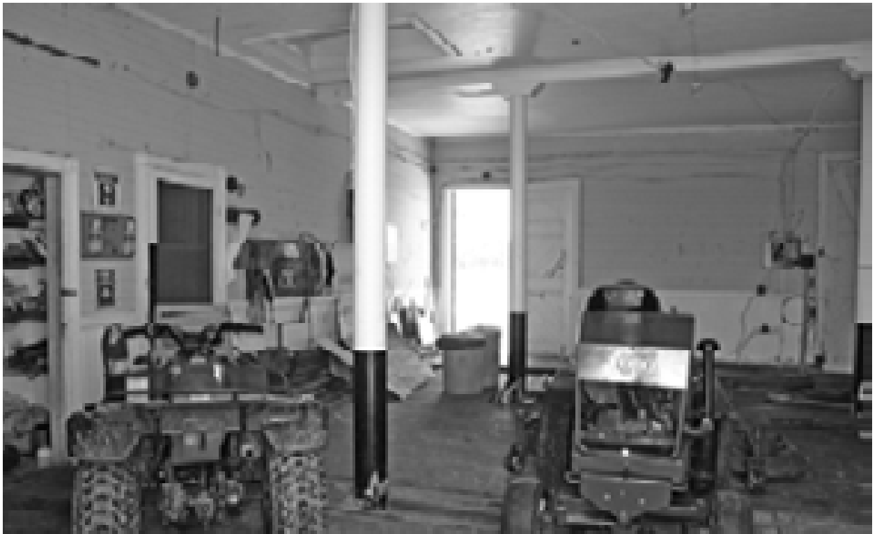
FIGURE 123. View west in Room 107. (T. Jones, NPS, 2005)
