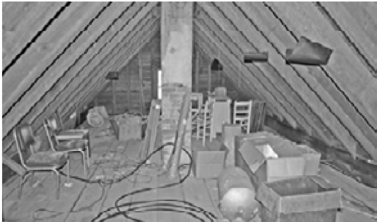
FIGURE 145. View southwest in attic. (T. Jones, NPS, 2005)
