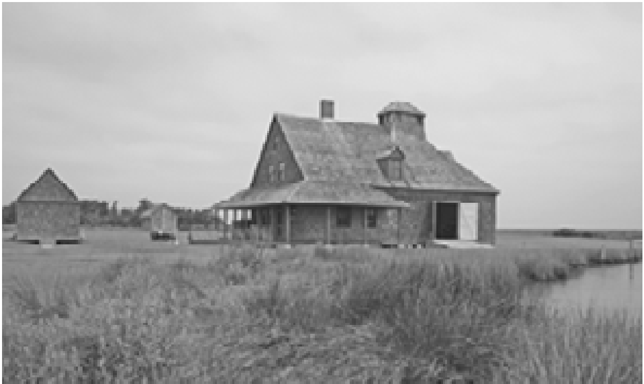
FIGURE 54. View north of Portsmouth Life-Saving Station, with kitchen at left and stable beyond. (NPS, 2005)
