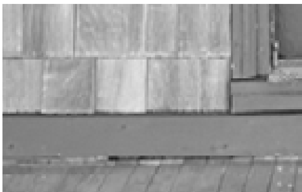
FIGURE 68. View of typical plinth at exterior walls. (T. Jones, NPS, 2005)
