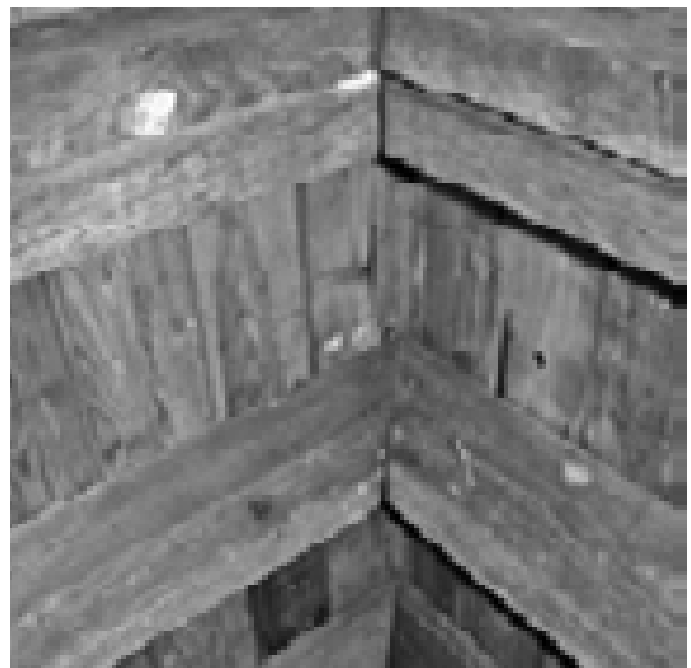
FIGURE 66. View at ridge of main roof. (T. Jones, NPS, 2005)
