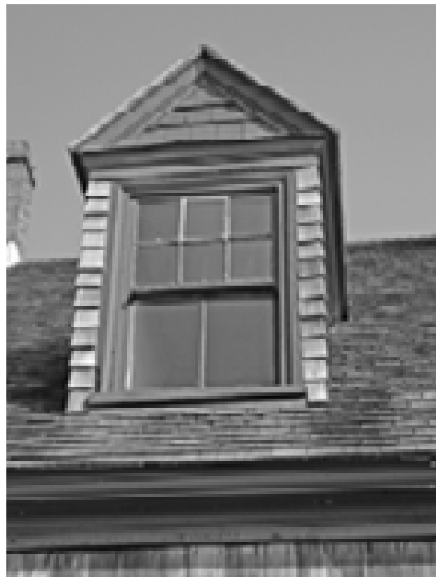
FIGURE 77. View of southeast dormer. (T. Jones, NPS, 2005)
