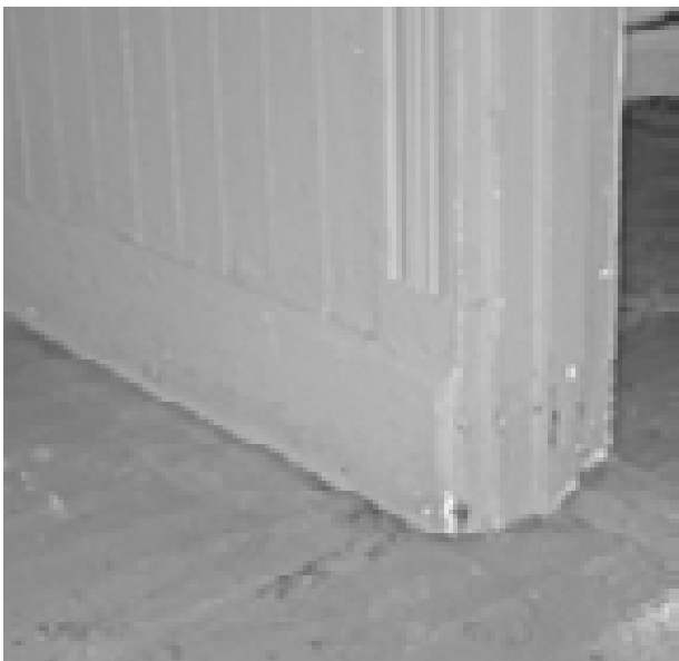
FIGURE 90. View of typical flooring, wainscot, and baseboard. (T. Jones, NPS, 2005)
