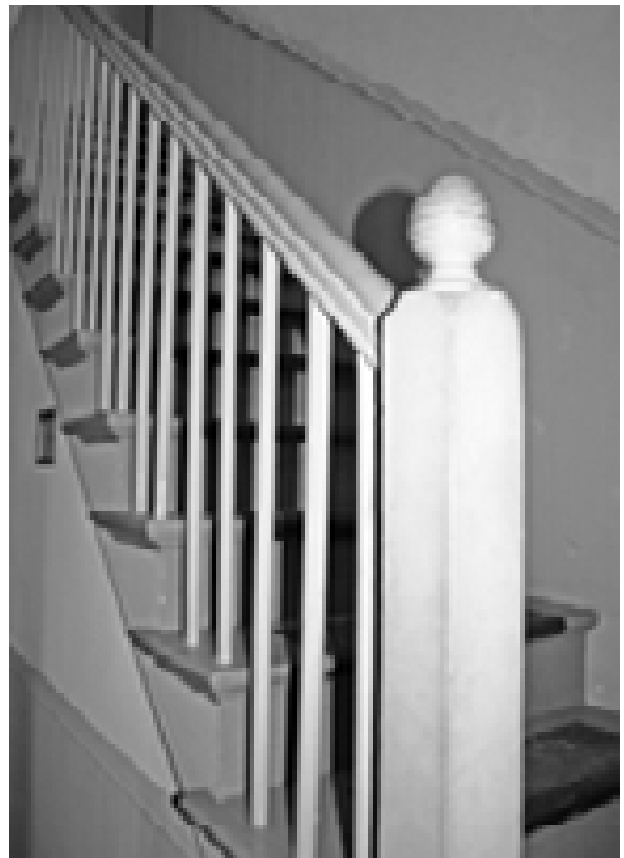
FIGURE 115. View of newel post and bannisters. (T. Jones, NPS, 2005)
