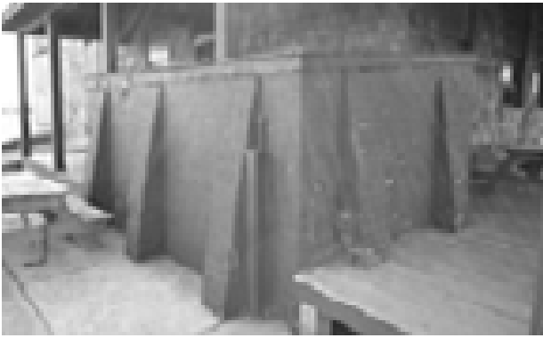
FIGURE 61. View east of cistern. (T. Jones, NPS,
