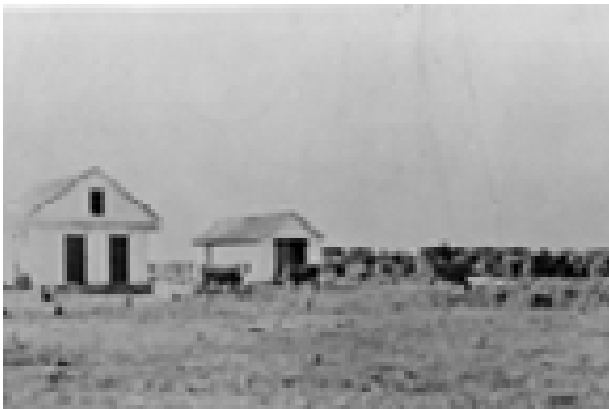
FIGURE 24. View of abandoned stables and boat house in 1946. (CALO Coll. A-46)
