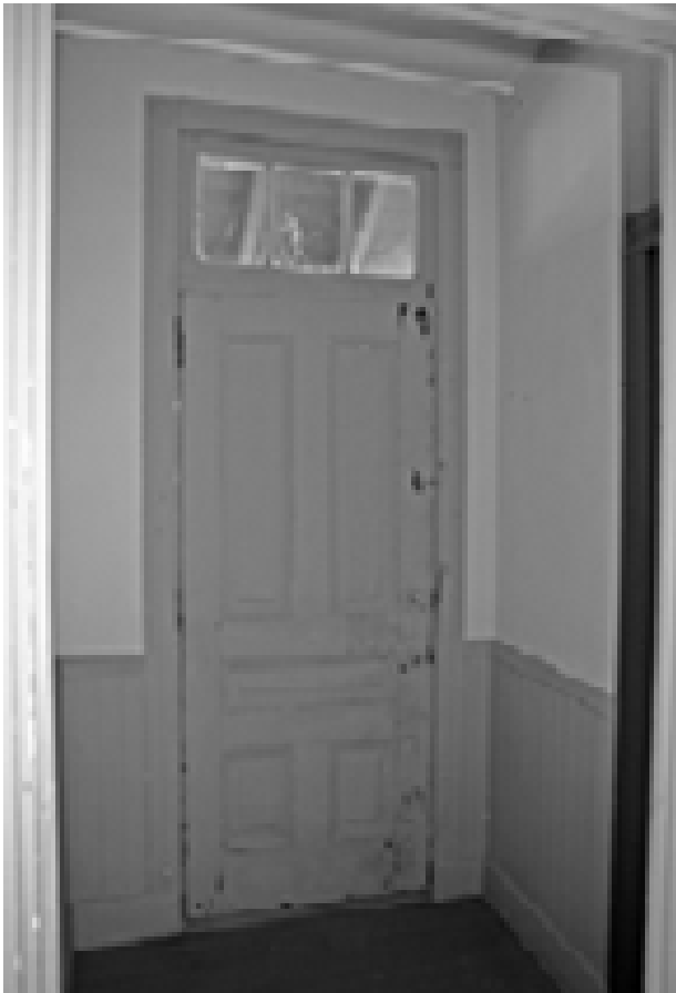
FIGURE 93. View north from Room 102 into Room 100. (T. Jones, NPS, 2005)
