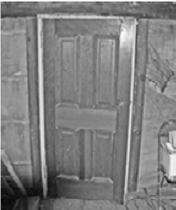
FIGURE 146. View of attic door. (T. Jones, NPS, 2005)
