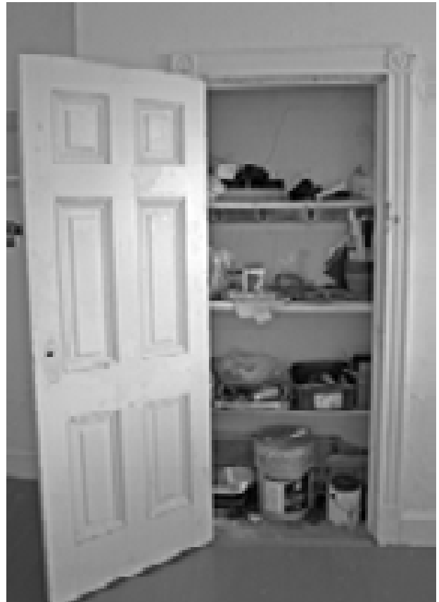
FIGURE 119. View of closet in Room 106. (T. Jones, NPS, 2005)
