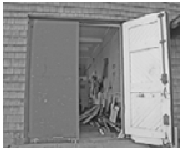
FIGURE 80. View of Door D-5. (T. Jones, NPS, 2005)
