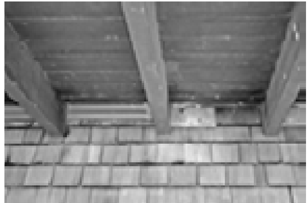
FIGURE 72. View of junction of porch rafters and walls. (T. Jones, NPS, 2005)
