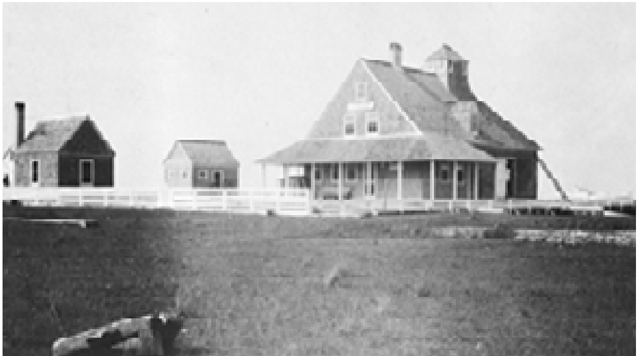
FIGURE 43. View north of Portsmouth Coast Guard Station, dated July 10, 1917. Barely visible at extreme left are the station stables, with the 1908 kitchen in the foreground and the 1894 oil house at center. (CALO Coll. A-67)
