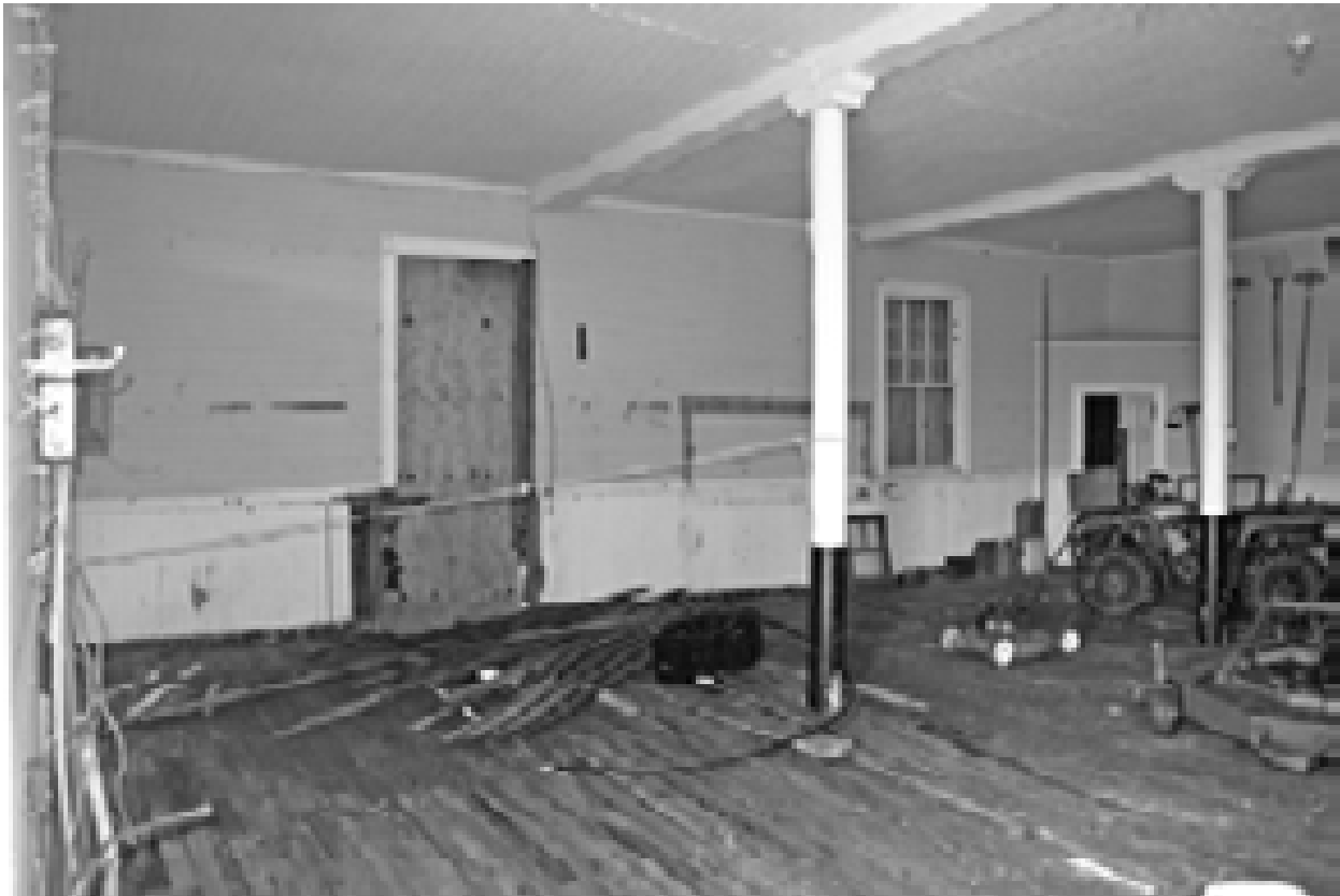
FIGURE 127. View east in Room 107. (T. Jones, NPS, 2005)
