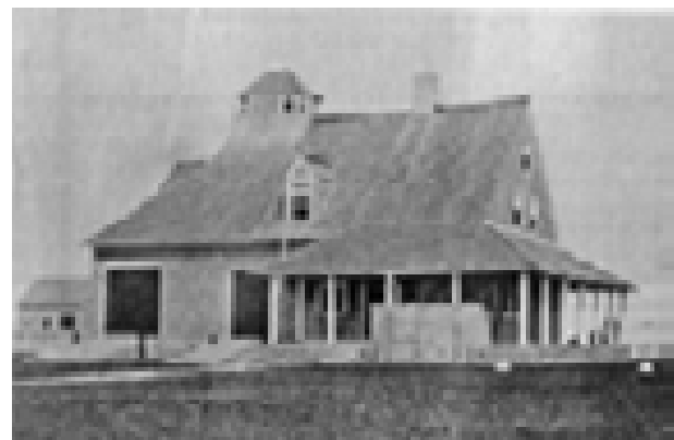
FIGURE 8. View of Core Bank Life-Saving Station prior to its expansion and remodeling in 1934. Note the stone foundation, which the Portsmouth station did not have. (CALO Coll.)
