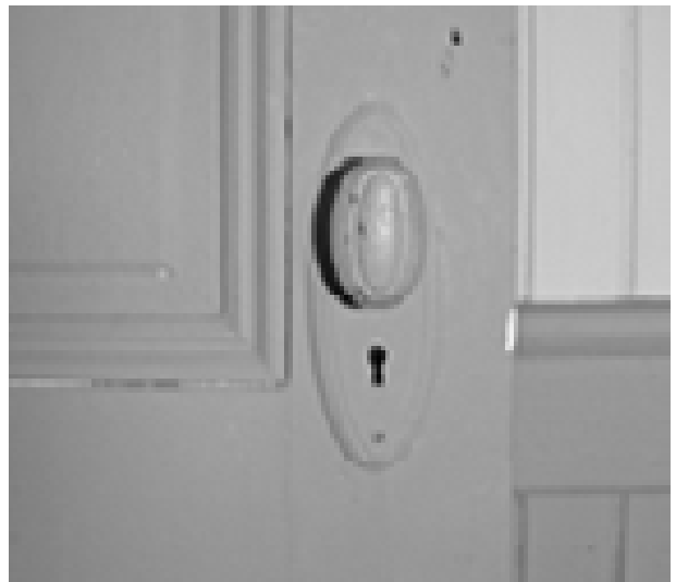
FIGURE 92. Typical door knob and escutcheon. (T. Jones, NPS, 2005)
