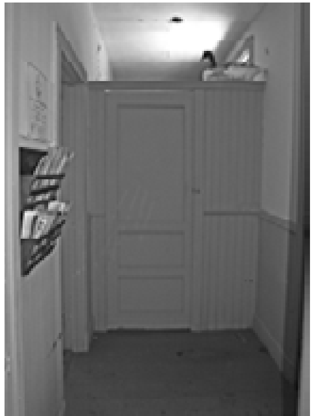
FIGURE 101. View southwest in Room 103. (T. Jones, NPS, 2005)
