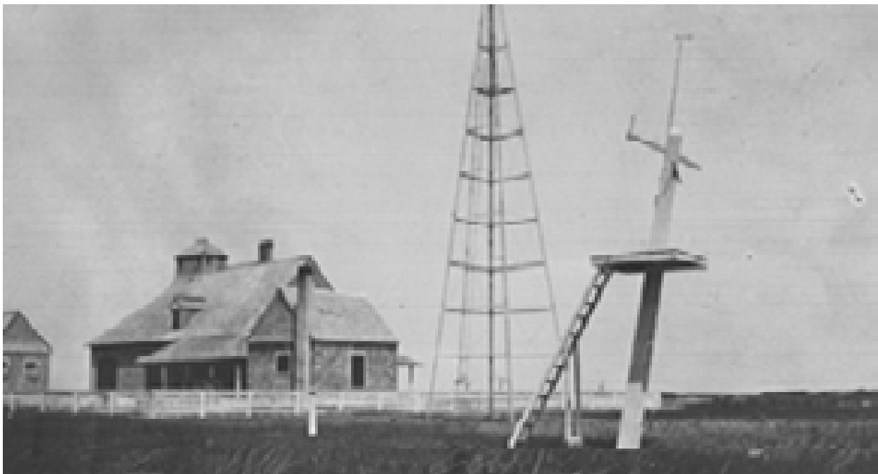
FIGURE 45. View east of station, 1916, one of few images showing the 1894 wreck pole, right, and the 1913 steel storm-warning tower. (CALO Coll. B-99)
