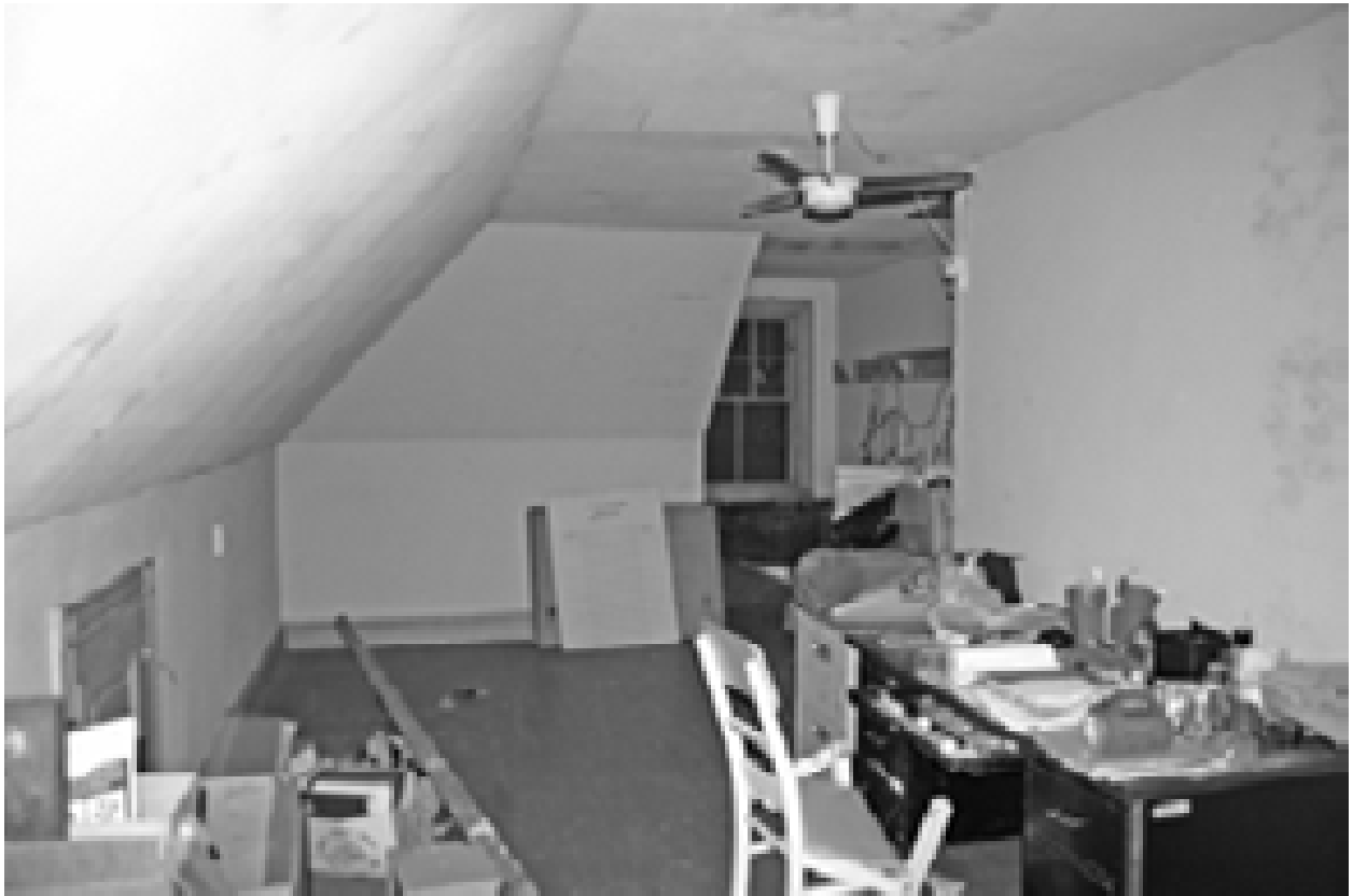
FIGURE 137. View northeast in Room 202. (T. Jones, NPS, 2005)
