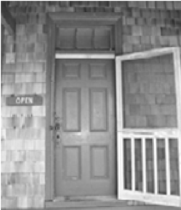
FIGURE 79. Door D-2 on southwest side of house. (T. Jones, NPS, 2005)
