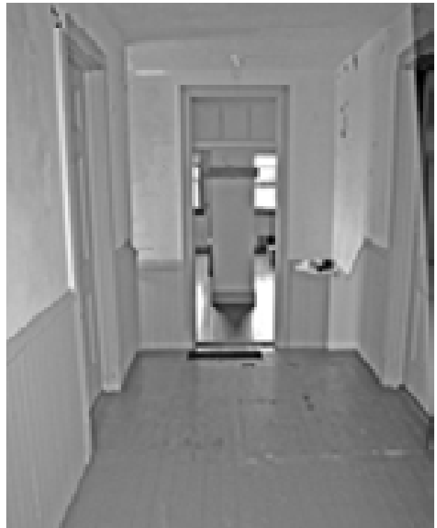
FIGURE 129. View southwest in Room 200. (T. Jones, NPS, 2005)
