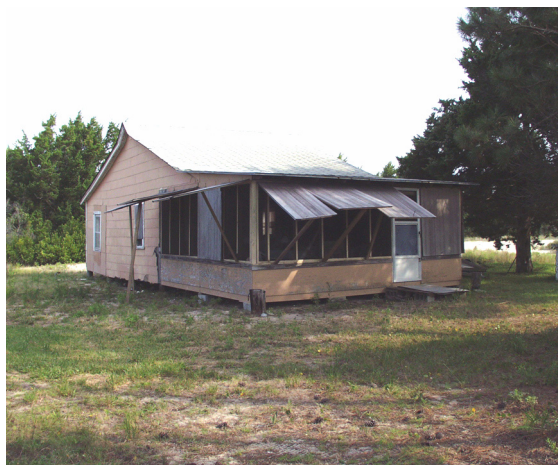
Figure 24 View to north of O'Boyle-Bryant House. (NPS-SERO-CRS, 2002)
