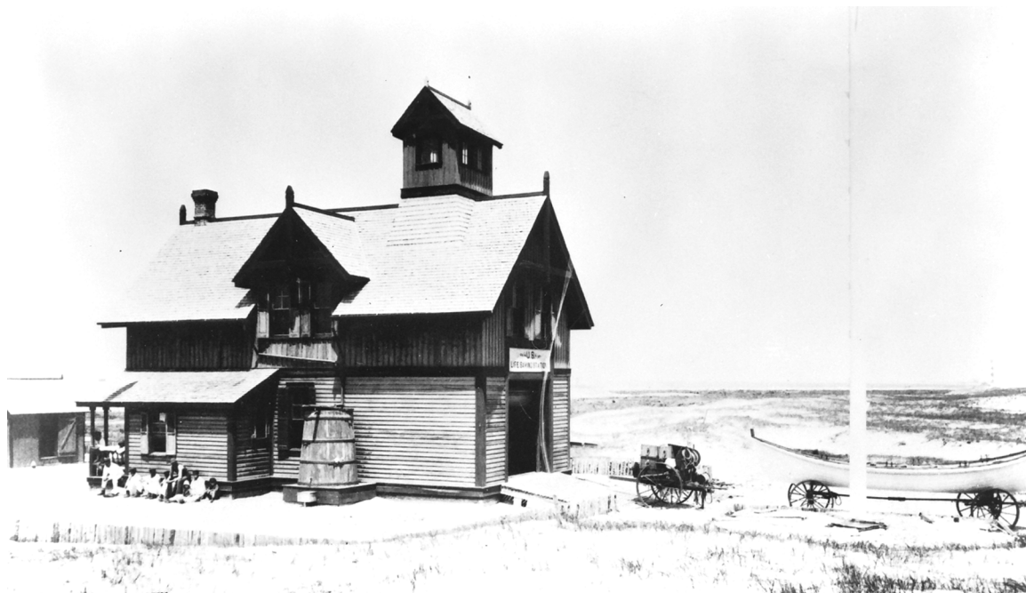
Figure 3 View north of the life-saving station, c. 1893, with the lighthouse barely visible on the horizon at extreme right. (CALO Coll. G-09)
