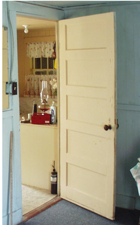
Figure 30 Five-panel door at Room 103. (NPS-SERO-CR, 2002)
