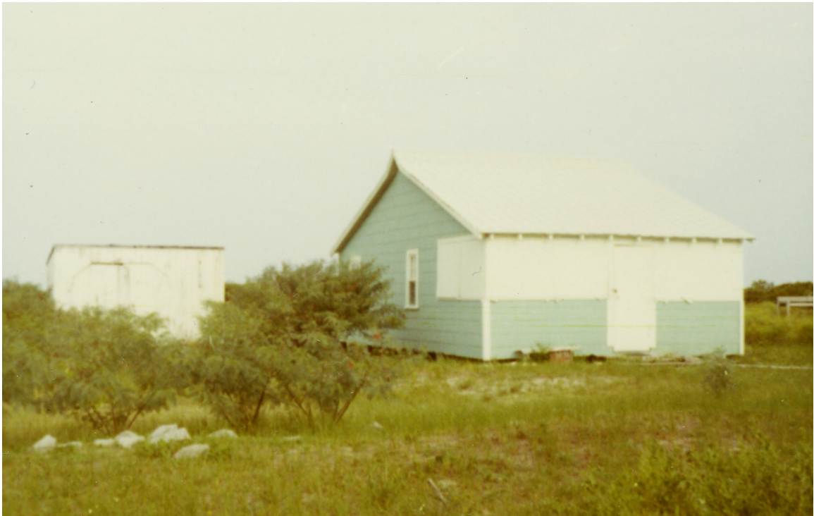
Figure 40 The goal of the proposed plan is a return of the house to its general appearance in this image, c. 1970, minus the asbestos siding. (CALO Coll., Phelps#6)
