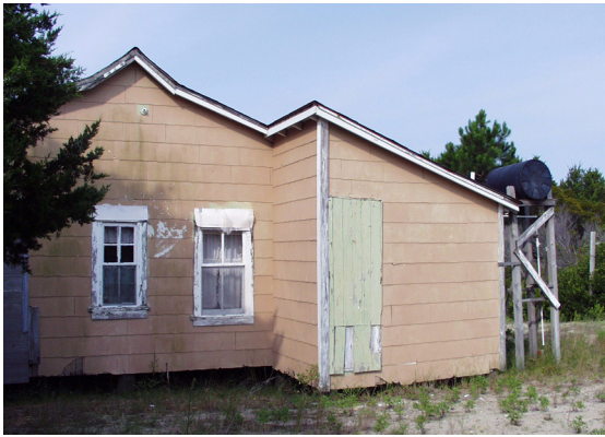
Figure 26 View of house from northeast showing bathroom addition. (NPS-SERO-CRS, 2002)
