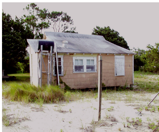
Figure 25 View to south of O'Boyle-Bryant House, showing elevated water tank. (NPS-SERO-CRS, 2002)
