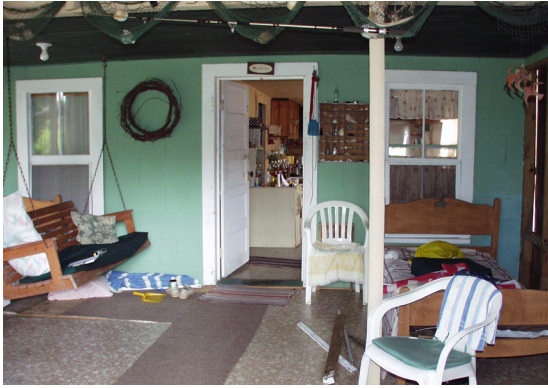
Figure 32 View of front porch. (NPS-SERO-CR, 2002)
