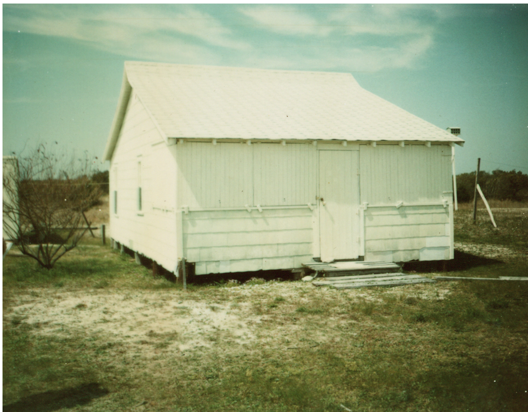
Figure 22 View of O’Boyle-Bryant House, 1976. (CALO Coll.)
