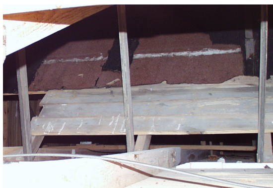
Figure 29 View of original (1939) asphalt roll roofing in attic. (NPS-SERO-CR, 2003)
