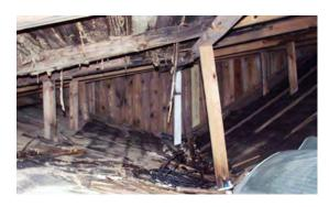
Figure 26 View of junction of roofs of two original structures; note severe termite damage in rafters and decking at left. (NPS-SERO-CR, 2002)
