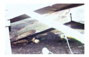
Figure 25 View of collapsing floor under Room 104. (NPS-SERO-CR, 2002)
