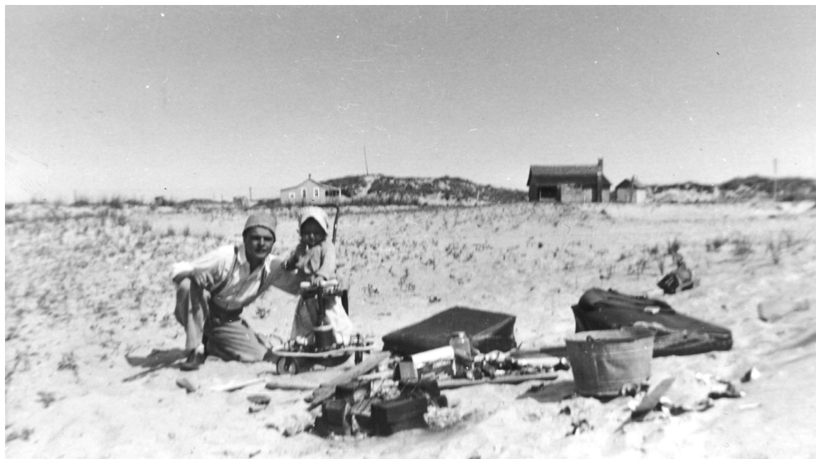
Figure 10 View to northeast from near Coast Guard Station, April 1941. (CALO Coll., O'Boyle #21)
