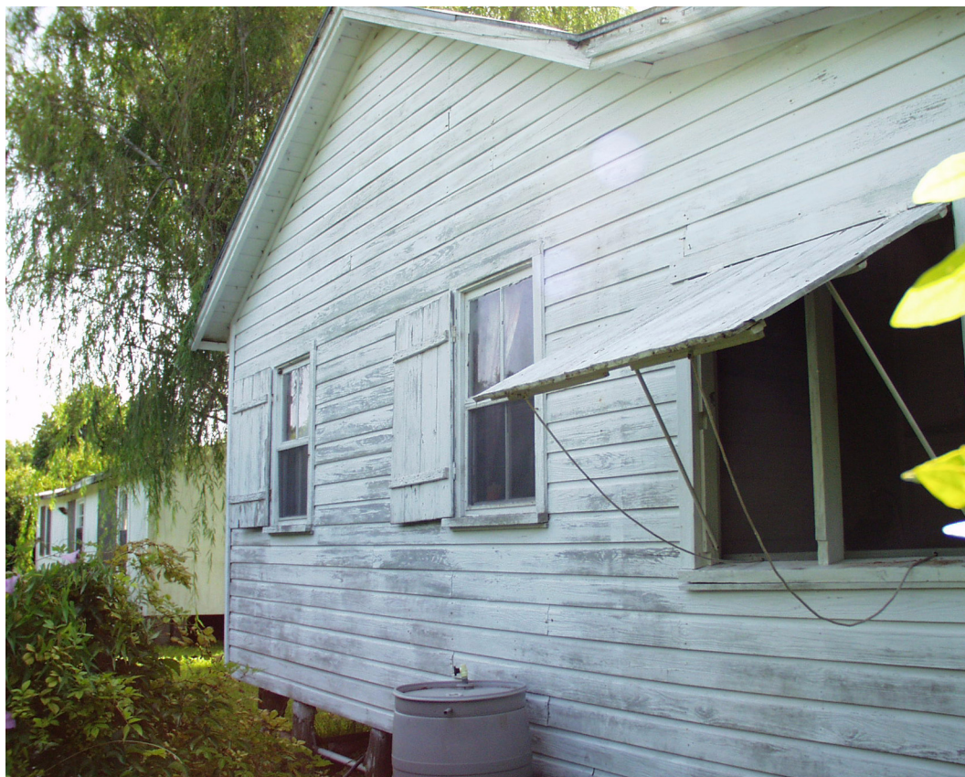
Figure 14 View east showing typical exterior finishes. (NPS-SERO-CR, 2002)
