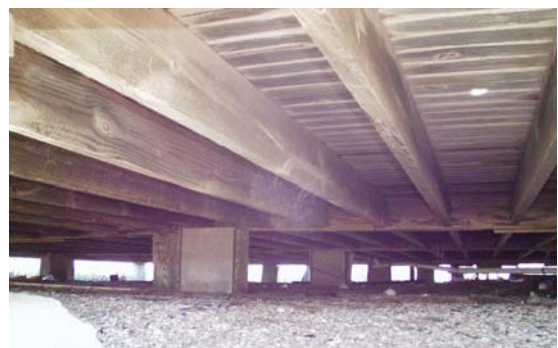
Figure 21 View of typical floor framing. (NPS-SERO-CR, 2002)
