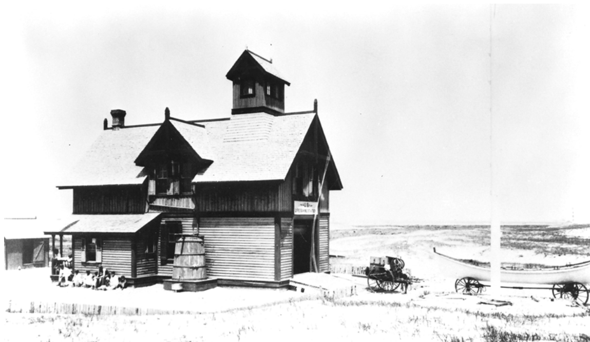
Figure 3 View north of the life-saving station, c. 1893, with the lighthouse barely visible on the horizon at extreme right. (CALO Coll. G-09)
