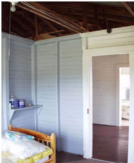
Figure 33 View north in Room 106. (NPS-SERO-CR, 2003)
