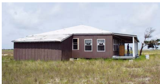
Figure 18 View of rear (southeast) side of house. (NPS-SERO-CR, 2002)
