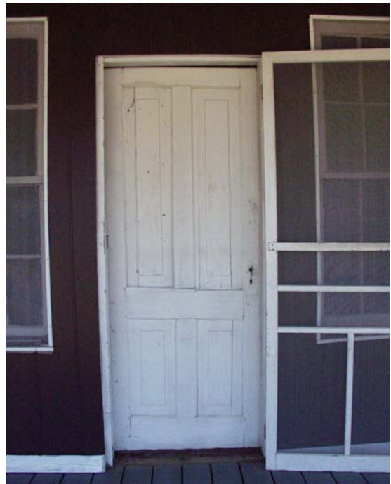
Figure 23 View of front door, which is presumed to be original. (NPS-SERO-CR, 2003)
