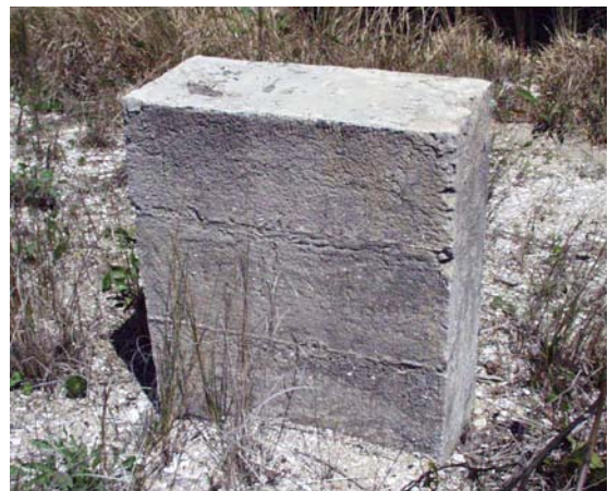
Figure 20 View of typical concrete pier. (NPS-SERO-CR, 2002)
