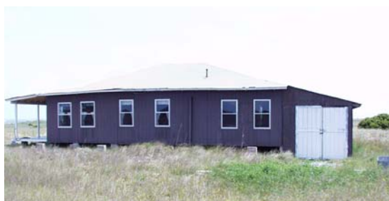
Figure 17 View of southwest side of house. (NPS-SERO-CR, 2002)
