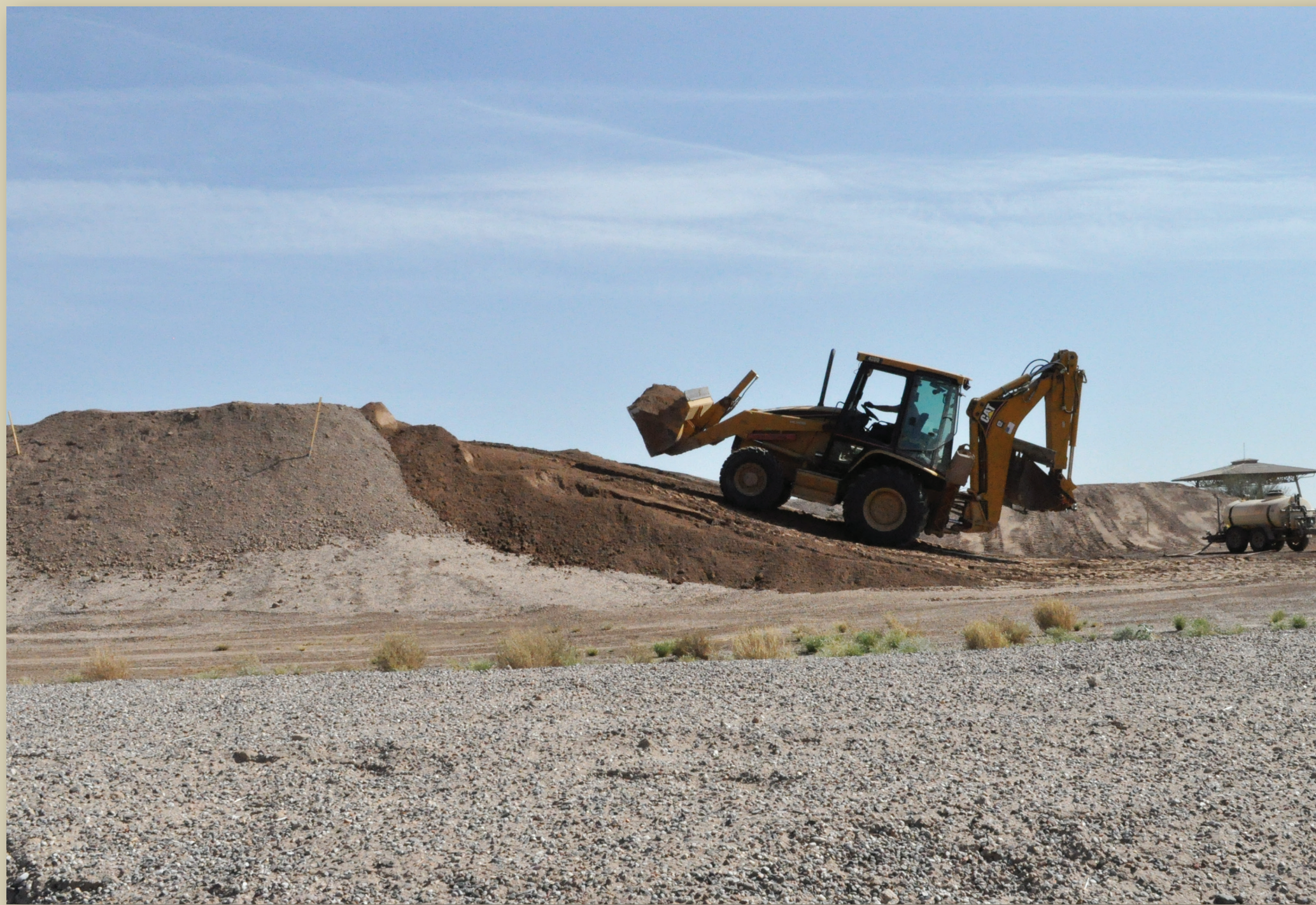
Backfilling involves reburying ruins with soil. This preservation method cannot stop deterioration, but it can slow down erosion and stabilize the site.
