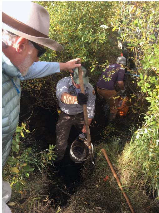
NPS staff and partners prepare a site for SBS installation.
