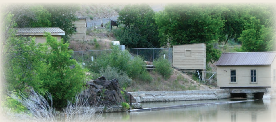
Gate and equipment houses provide for the workings of the tunnel at East Portal. NPS
