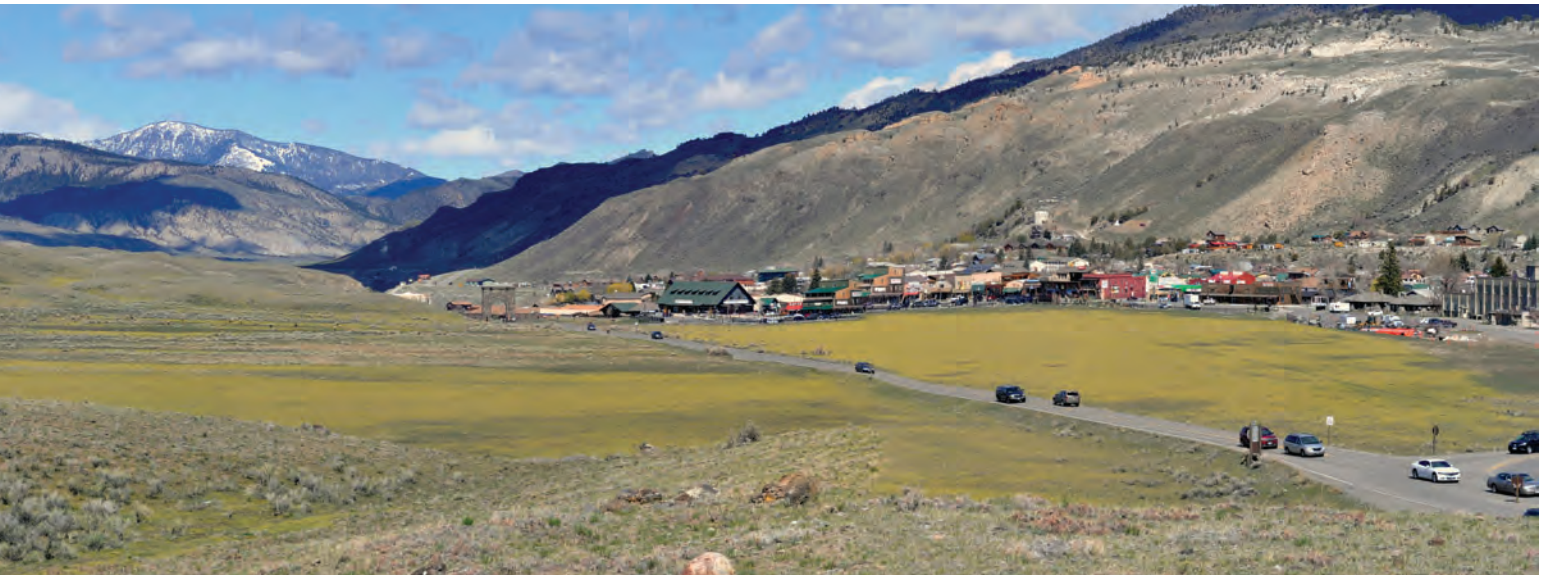
NPS PHOTO: S. WACKER
