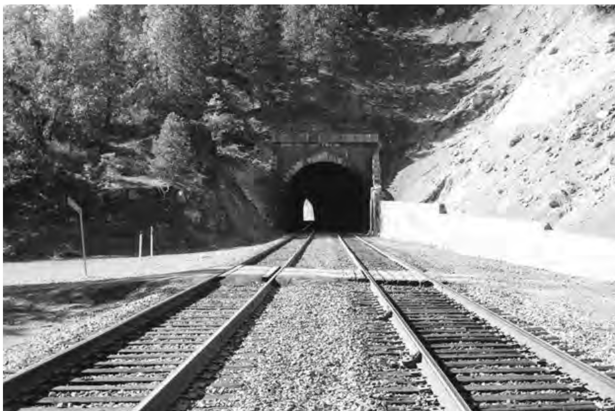
East Portal of Tunnel 1, Central Pacific Railroad, Placer County, California. Chinese workers made tremendous contributions to railroad construction, particularly tunnels. This tunnel was built in 1868. HAER photo by Ed Anderson, courtesy of the Library of Congress.
