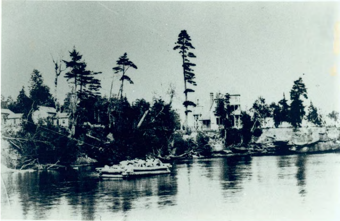
Figure 21. Excelsior quarry on Hermit Island, workers' houses on left, Cedar Bark Cottage on right, 1890s. Courtesy of Apostle Islands National Lakeshore.
