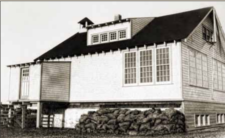
Photo 24. Attu schoolhouse. (Source: UAF Historical Photograph Collection, Vertical File Photograph Collections-Towns-Attu)
