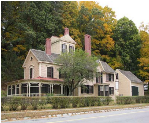
The Wayside, a National Historic Landmark in Minute Man NHP
