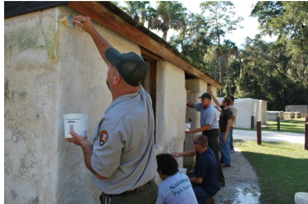
Limewash workshop on tabby cabins at Kingsley Plantation in Timucuan Ecological and Historic Preserve.
