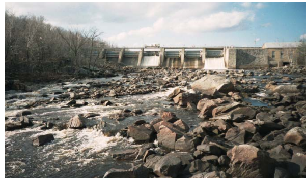
Existing bypass reach below Grandfather Falls Hydro Project is location of potential future enhanced flows for whitewater boating and aquatic ecology enhancement.
