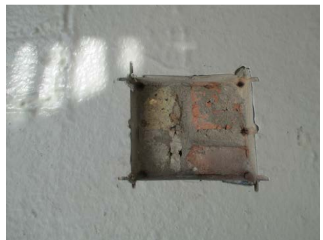
Stucco core sample from the Addison Street wall.
