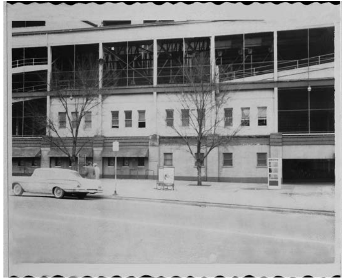
Early-mid 1960s photo showing the partial removal of the clay tile roof and complete removal of the ornamental grilles.
