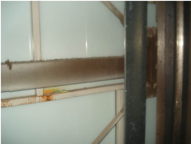
5. Clean down hoistway
