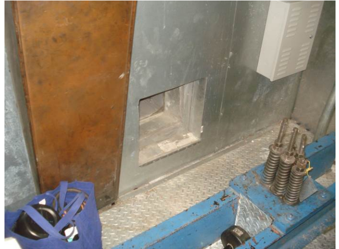
14. Provide covers on A/C vent
