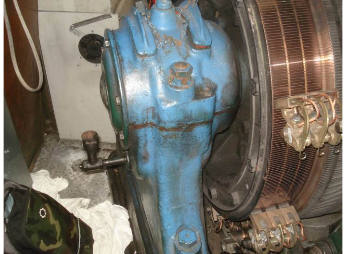
2. Clean hoist machine of accumulation of dirt
