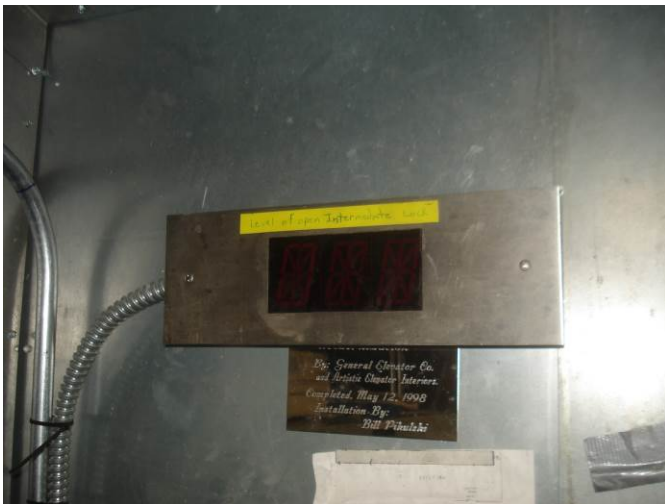
19. Repair position indicator in machine room
