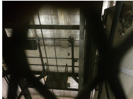
Figure 2: Elevator Access Platform at an Intermediate Level
