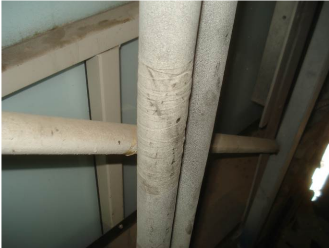
9. Confirm the traveling cables do not have shorts in the wires as there is tape on the traveling cable at the top and bottom of the hoistway
