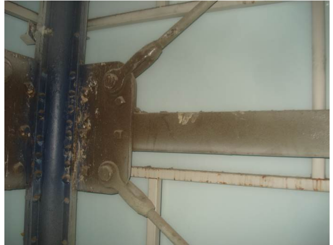
22. Clean inside hoistway of dust, dirt and debris
