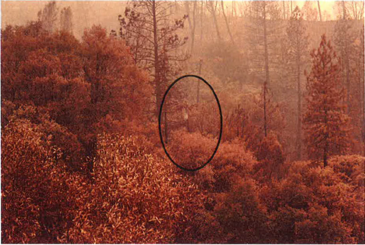
Photo 10 IMG_0765 South Power pole with hardware south of Highway 299W. Area was not burned on 7-23-2018.
