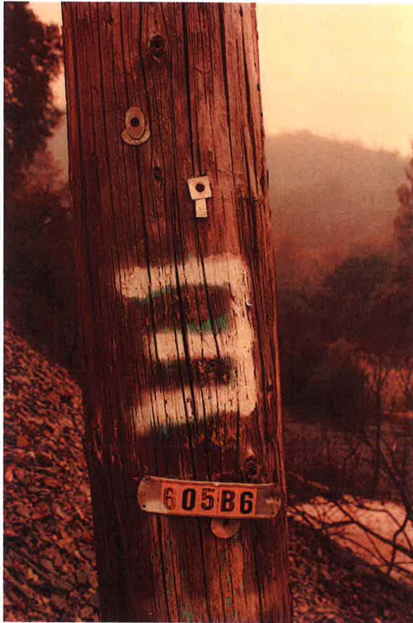
Photo 13 IMG_0768 Fire B Closeup of power pole #605B6
