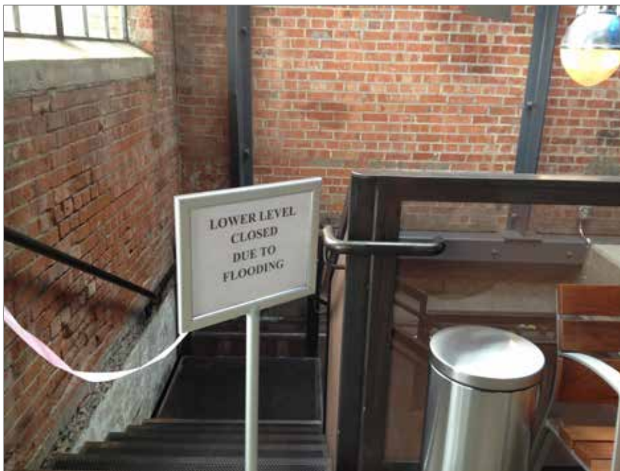
Photo 2. Basement flooding in the visitor center at Rosie the Riveter WWII Home Front National Historical Park. This photograph was taken on December 5, 2012 —12 years after the establishment of the park. Photo credit: Maria Caffrey.
