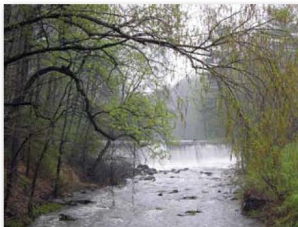
Burnt Mills Dam, Maryland.
