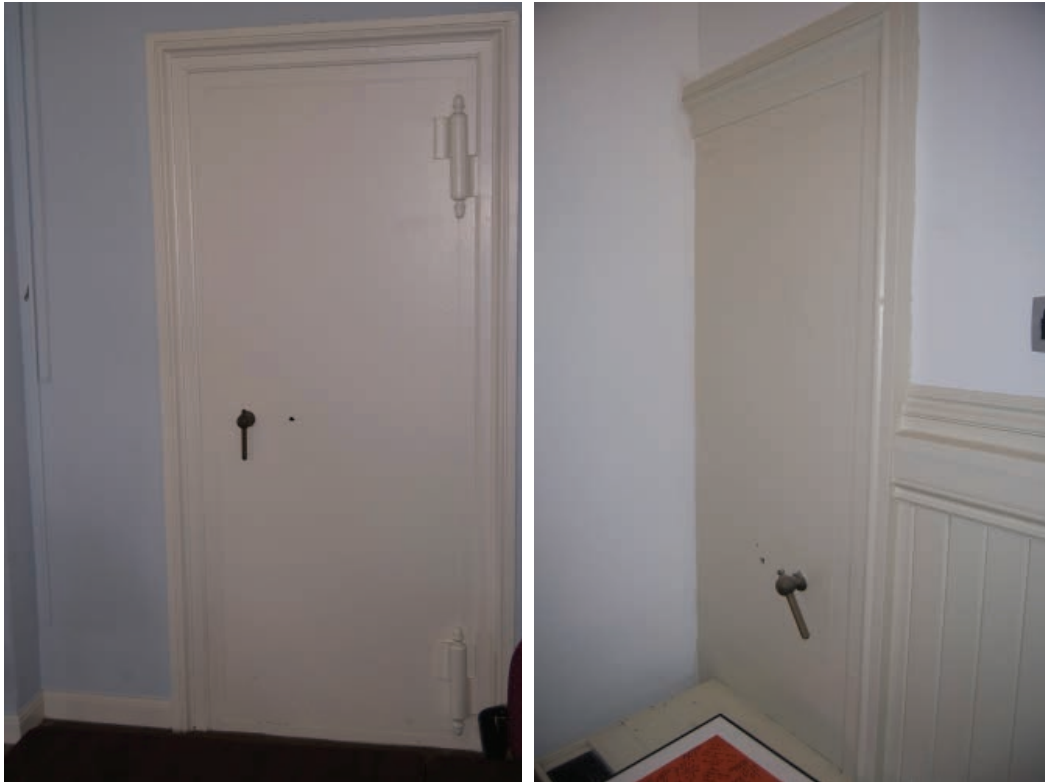
Photo # T-160 and # T161 Typical vaults and vault doors located at selected offices in the Old Post Office. See schedule to the right for locations.
