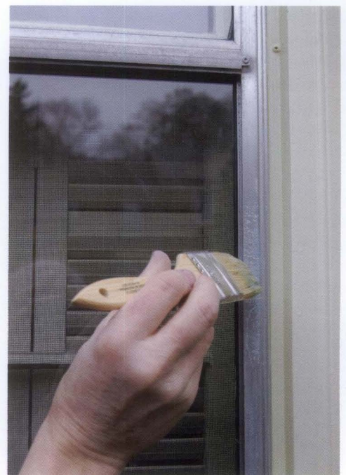
Figure 12. Cleaning tests may include a variety of products and methods such as mild soaps and detergents, etching cleaners, and abrasives. The gentlest means possible should be used, understanding that the goal is not to create a like-new appearance but rather to remove excessive grime and surface pollutants. Use of heavy etching cleaners or heavy-duty abrasives should be avoided on certain historic finishes. In this photograph a mild etching cleaner in jell form is being tested on a storm window with a mill finish.
