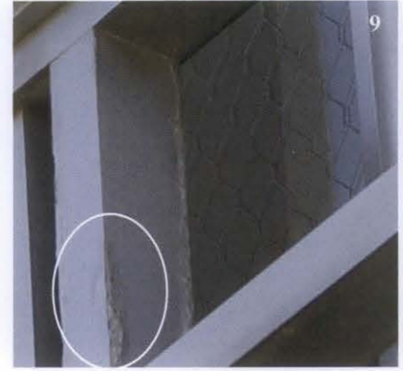
Figures 7 and 8. Aluminum corrosion can appear as a white discoloration and forms on the surface as the protective oxide film breaks down, as seen in these 60 year old windows in the PSFS Building, Philadelphia, before they were replaced. The small dark bumps are where surface dirt, grime, and pollution particles collect. Over time, pits form beneath these dark areas as the surface continues to corrode. This corrosive action is further encouraged by foreign particles, such as dirt and chlorides, which hold moisture next to the surface. (Photo: Powers & Company Inc.) Figure 9. Some aluminum alloys are less corrosion resistant than others. Delamination, as seen on this aluminum railing in front of a window at the Folger Shakespeare Library, can occur when an aluminum-copper alloy is introduced and used in an outdoor setting. The original specifications called for aluminum and chromium, but were not followed.
