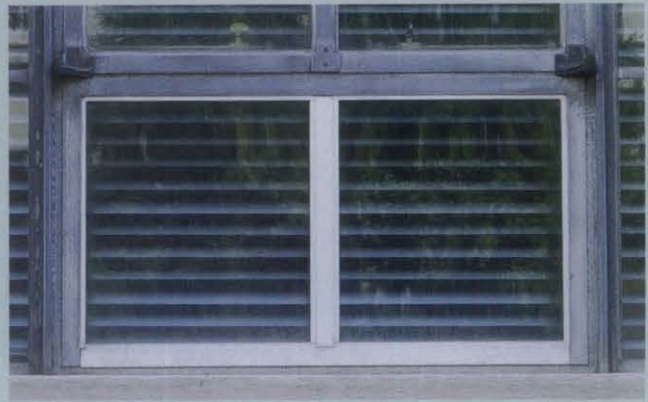
Figure d. Numerous hopper units have been removed over time to accommodate air conditioning units. Replacement hopper units were manufactured, as needed, to match the original hoppers elsewhere in the building.
