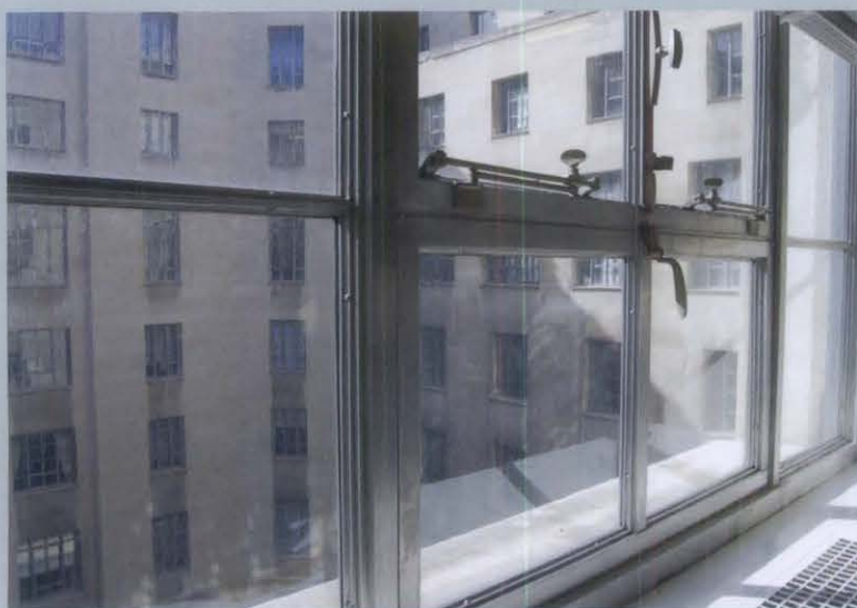
Figure c. In cleaning historic aluminum windows, the gentlest means possible should be used. More aggressive cleaners should be used only where necessary. The interior surface of this window was cleaned ten years ago with an aluminum jelly cleaner, rinsed and then dried thoroughly. The original mill finish still retains its luster.
