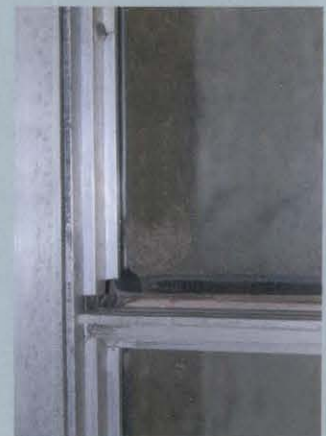
Figure b. The panes of glass were secured into the frame with aluminum glazing stops, each individually cut, drilled, and fixed in place from the inside. Here the vertical stop is in place while the horizontal is missing.
