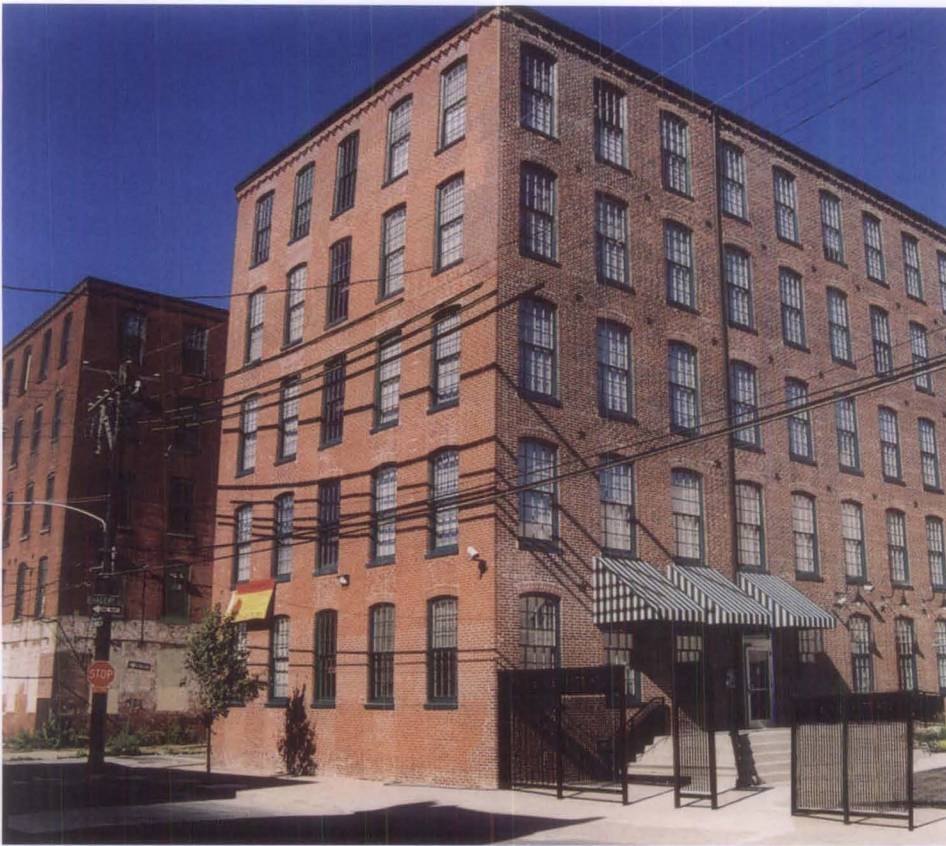
Figure 8. Upon completion of the work, the former mill now serves as low-income housing and artist live/work space. The new wood windows provide improved energy performance and enhance the visual qualities of the historic building.
