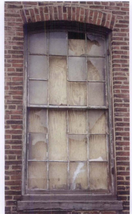
Figure 2. The historic double-hung wood windows had narrow sash and frame members that contributed to the distinctive qualities of the windows.
