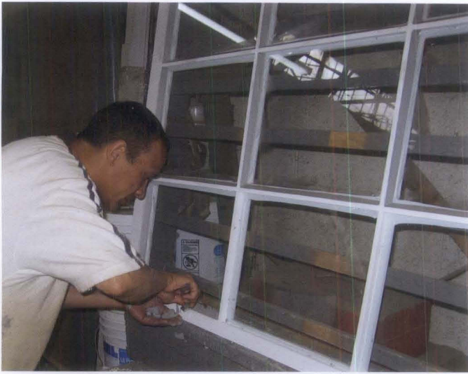
Figure 6. The outer glass was installed in the traditional manner, using exterior glazing putty. Photo: Charles Fisher.
