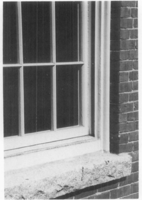
Figure 7. The retention of the exposed outer face of the historic wooden frame and the sill detailing were important qualities of the window treatment. Before and after photos: Charles Parrott
