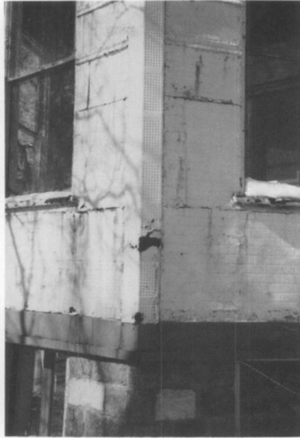
4. Rust stains indicate where corrosion, caused by water infiltration, are breaking through the metal from the rear. Rust and separation are also evident at seams between sheets of stamped metal. Inspection determined that nearly 90% of the stamped metal siding had to be replaced. Photo: Richard Hiler.
