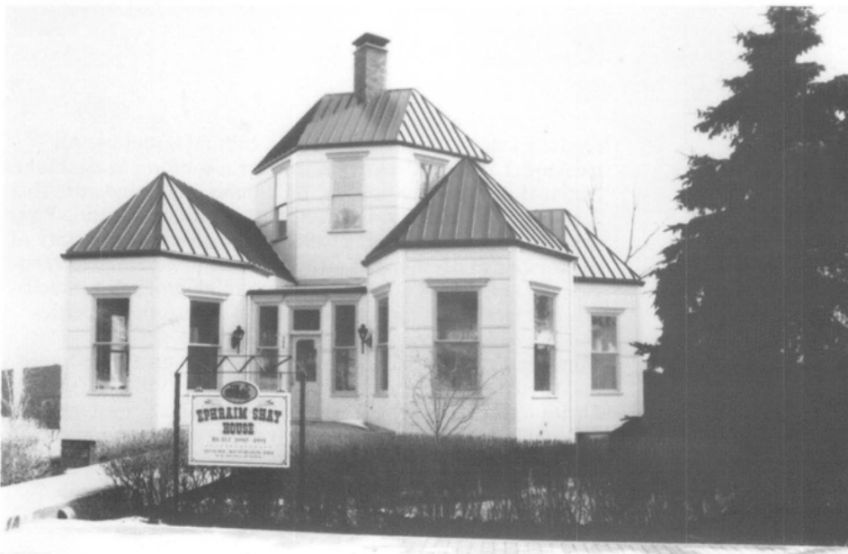
12. The replication of the stamped metal siding has restored the Hexagon to its historic appearance. A new metal panel roof system that duplicates the appearance of the original standing seam roof also contributes to the restoration. Photo: Richard Neumann.
