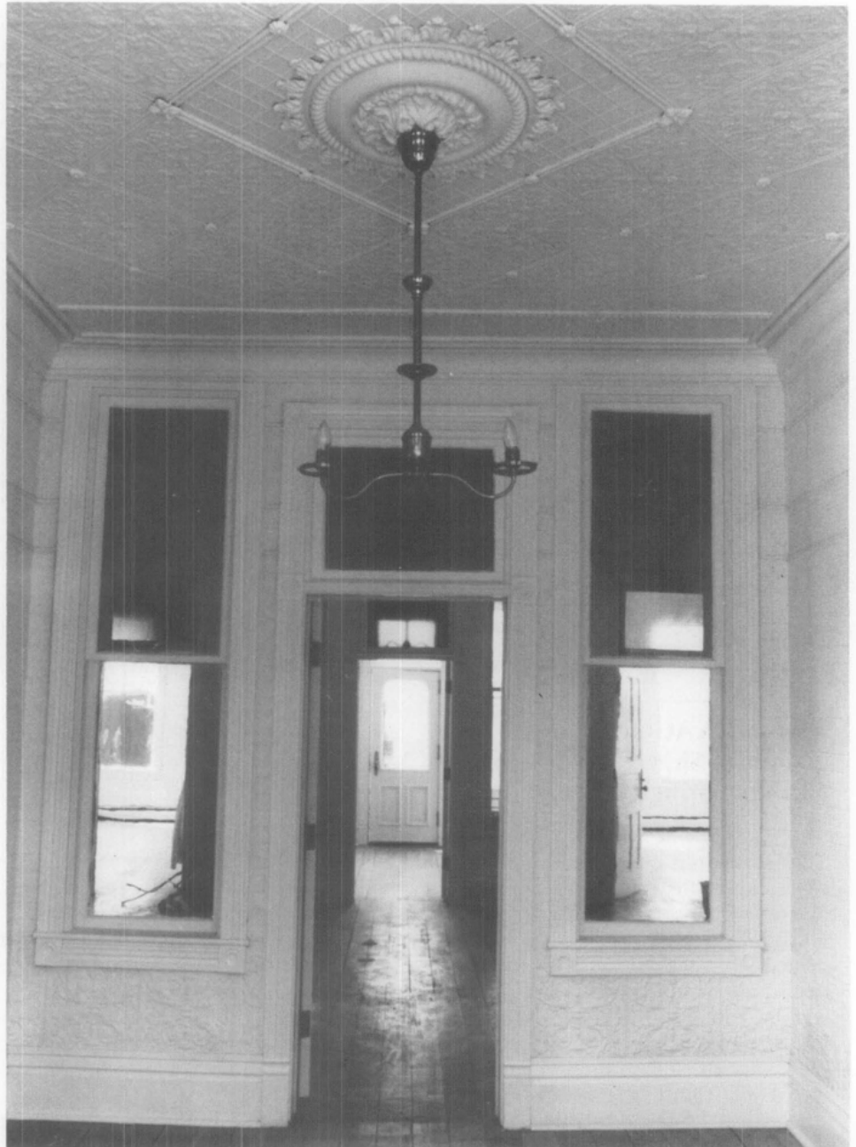
2. The walls and ceilings of each interior room are sheathed with stamped metal siding in a variety of decorative patterns. Photo: Brian Conway.
