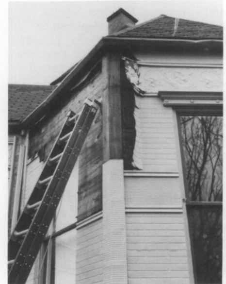
9. Original exterior siding was removed, revealing the exterior plank wall sheathing, which was also removed in order to install additional insulation and a vapor barrier. Photo: Mary Cay Bartush Jones.
