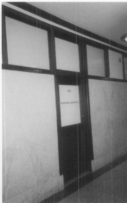
Figure 10. Completed Fisher building corridor with back painted door and tripartite transom. Photo: National Park Service File.
