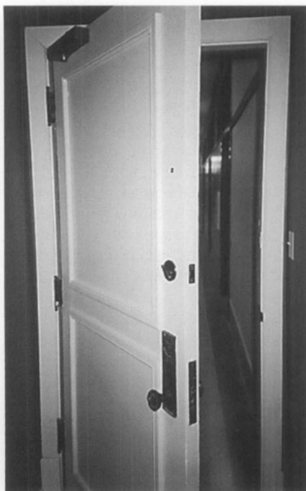
Figure 9. Fisher Building door viewed from apartment showing gypsum board infill panels, new trim and retained hardware. Photo: National Park Service File.
