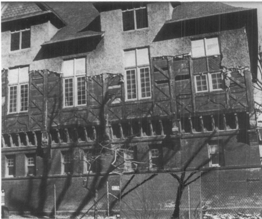
Figure 1. The stucco, applied circa 1910, is shown here being removed as part of the 1980 restoration. The wooden siding and "half-timbering" was largely intact underneath. Photo: Courtesy of Gallaudet College
