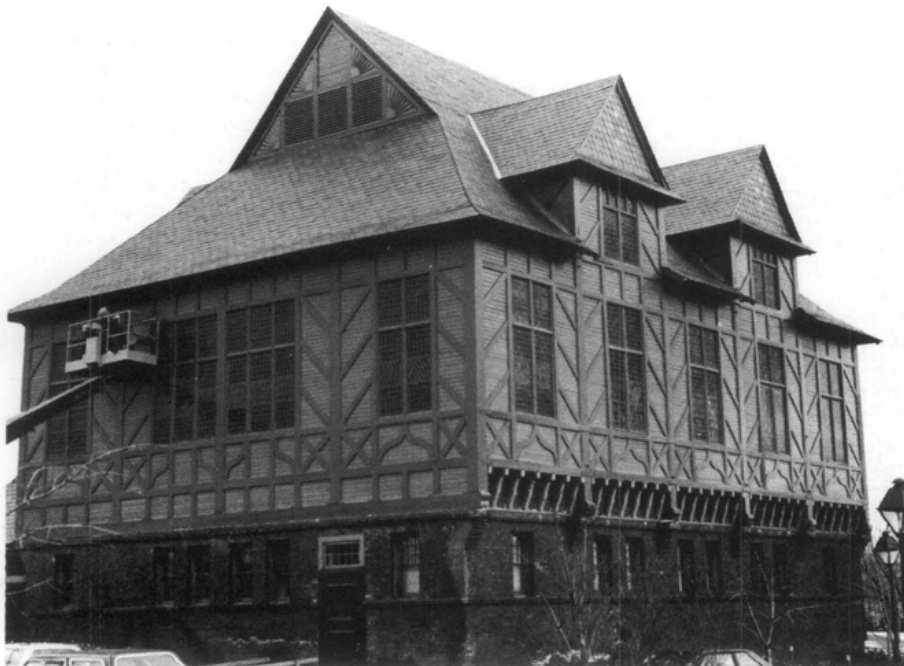
Figure 10. The college will inspect the building on a regular basis to ensure that any problems are immediately corrected. Photo: Charles Fisher
