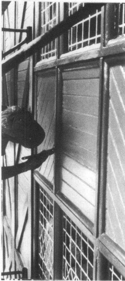
Figure 9. The building was painted with two coats of oil-alkyd primer and two top coats of acrylic latex. Photo: Bryan Blundell
