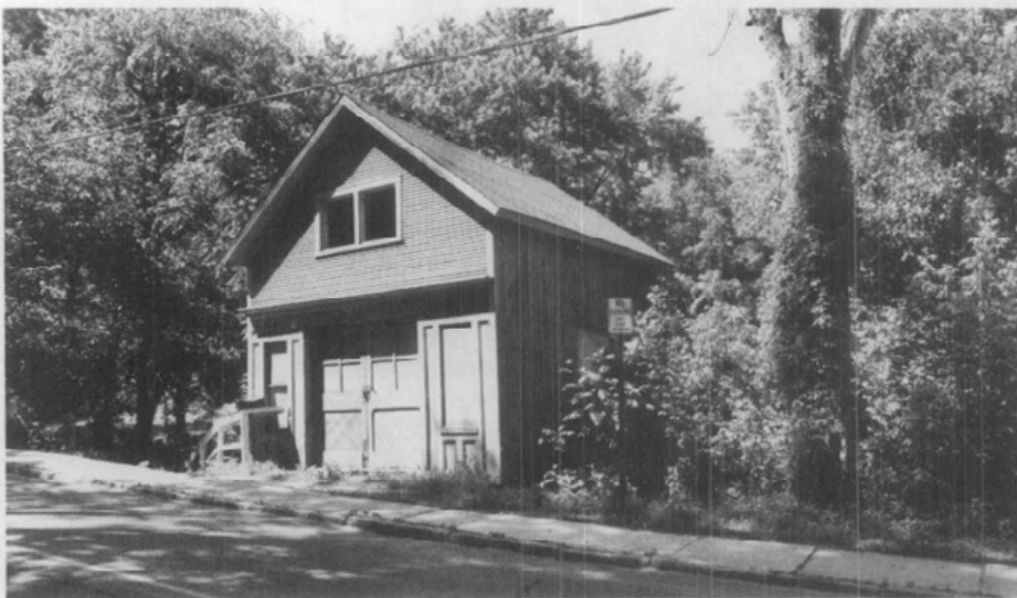
Figure 8. This 1870s carriage and wagon painters shop never had a customers' entrance other than through the carriage doors. Photo: Charles Fisher
