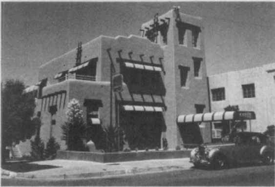
Monte Vista Fire Station
