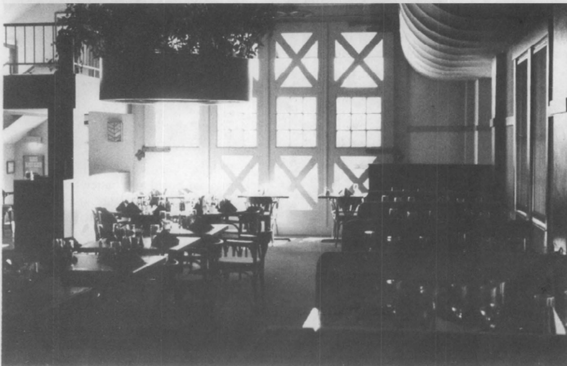
Figure 7. Replacing the tongue-and-groove boards with glass opened up the former fire truck bay while retaining the character of the doors.
