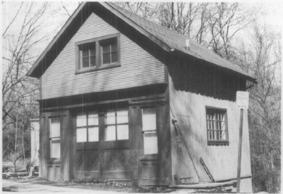
Figure 9. A new customer entrance was created through construction of a door along the side. The concealed nature of the door minimized its impact on the building's historic appearance. Photos: Charles Fisher
