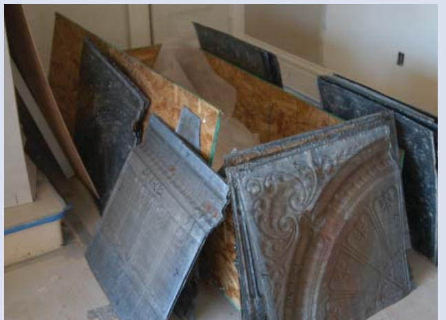
Figure c. Once the metal was cleaned of over 100 years of paint, it was easy to see the detail of the original design.
