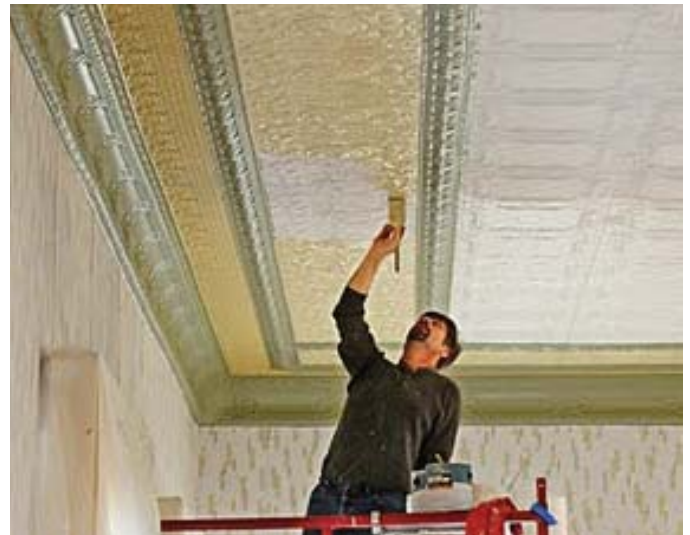
The historic polychrome appearance is being recreated and enhances the depth and complexity of the decorative metal ceiling. (Photo: The Madison Courier)
