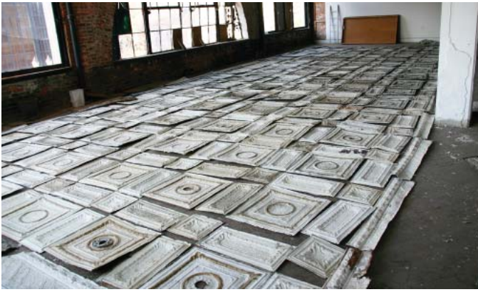
When carefully removing the historic pressed metal from the original ceiling above, the pieces were numbered and later arranged on the floor in the same way they appeared on the ceiling to aid in their reinstallation. (Photo: NPS file, 423 N Market St., Wilmington, DE)
