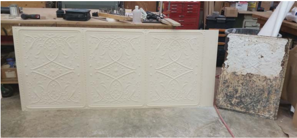
Another option for the replacement of individual tiles that may be irreparable in a field of otherwise salvageable material is digital replication. Through the careful removal of the tile, a skilled artisan can measure the exact dimensions and create a digital copy. Once an acceptable model has been created, the design can be replicated on a suitable substrate as shown. (Photo: Lonnie Coulter, La Bastille)
