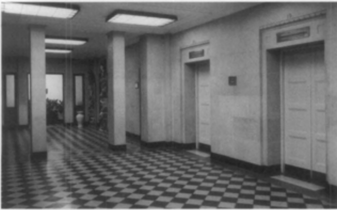
Figure 13. Quarry tiles were used in the corridors on many of the upper floors of the U.S. Department of the Interior Building (1935-1936). They were laid in a pattern identical to the more expensive marble floor tiles that were used in the public spaces. Photo: Brooks Photographers, HABS Collection.
