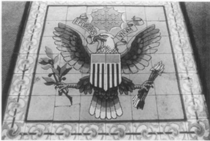
Figure 4. The tiled Presidential Seal in the courtyard of the Pension Building (now the National Building Museum), Washington, D.C., was installed in honor of President William McKinley's second inauguration in 1901. The "heavy Damask design," resembling fabric, that was used to decorate the tiles, indicates they were probably manufactured by The Mosaic Tile Company, Zanesville, Ohio, which first introduced this design. Photo: Kimberly A. Konrad.
