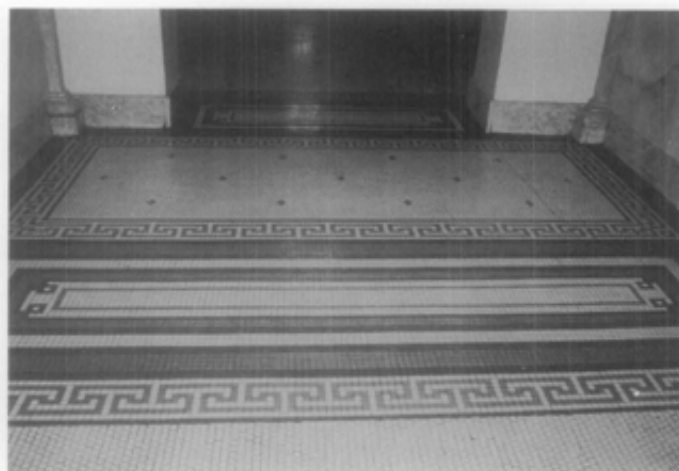
Figure 11. Ceramic mosaic tiles were used decoratively on the entrance floor of this early-20th century school building. Photo: Kimberly A. Konrad.
