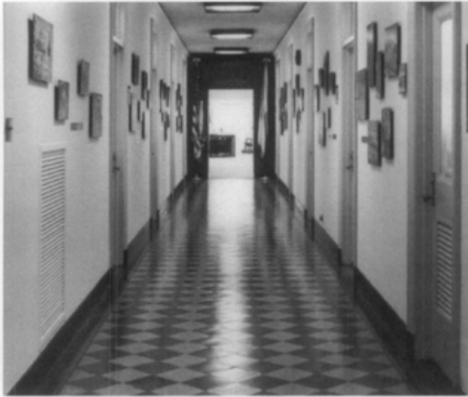
Figure 19. Regular maintenance treatments for the historic quarry tile floors in the U.S. Department of the Interior, shown here in a side corridor, include: stripping and waxing once a year; weekly spraying and buffing with a commercial "floor finish revitalizer/cleaner" that is slip resistant; and dust mopping or damp mopping 4 times a week. Photo: Brooks Photographers, HABS Collection.
