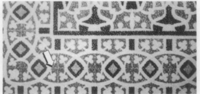
Figure 18. One-piece tiles were made with a mold that created the appearance of mortar joints and individual mosaics, as illustrated in Decorative Tile Designs in Full Color . Selected and arranged by Carol Belanger Grafton. NY: Dover Publications, Inc., 1992, p. 87.
