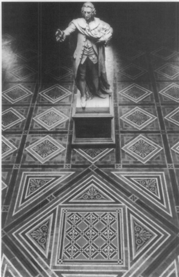
Figure 1. Minton encaustic tile floor, 3rd floor, Patent Office Building (now the National Portrait Gallery), Washington, D.C. Originally constructed between 1836–40 under the supervision of Robert Mills, the upper floors of this portion of the building were restored and redecorated in 1877 in the “Modern Renaissance style” by Cluss & Shulze, Architects, after a disastrous fire. Photo: Jack E. Boucher, HABS Collection.
