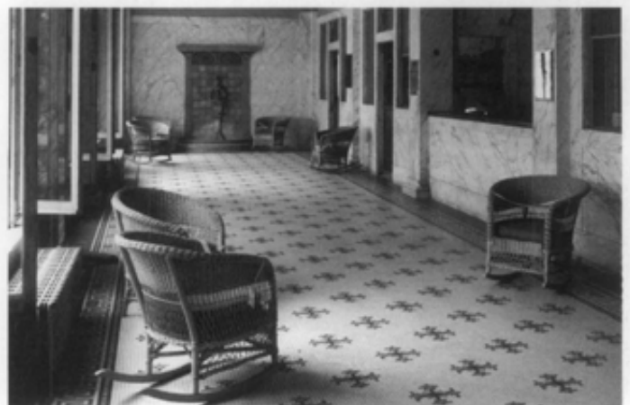
Figure 10. Ceramic mosaic tile floors were practical for structures like this Bath House, Hot Springs, Arkansas (1914-1915). Photo: Jack E. Boucher, HABS Collection.
