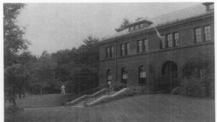
(d.) Hunnewell Visitors Center's entrance following rehabilitation, integrating an accessible path (left), platform, and new steps. Photo: Charles Birnbaum.
