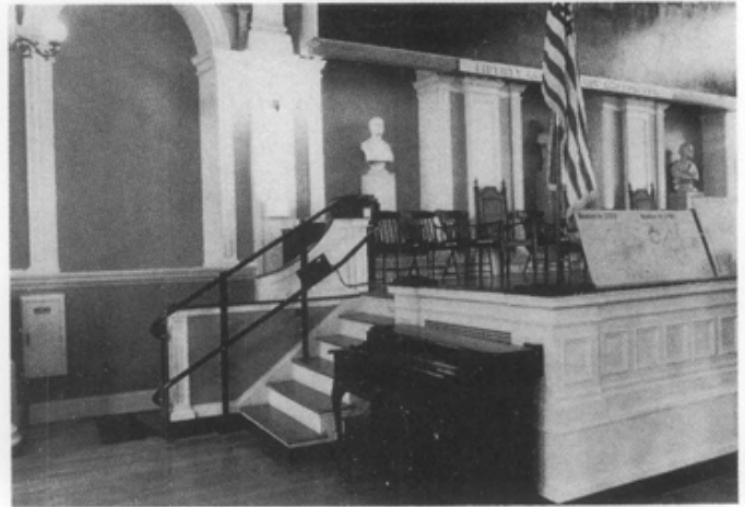
Figure 19. Inclined lifts can sometimes overcome interior changes of elevation where space is limited. This lift in Boston's Faneuil Hall created access to the floor and stage level of the State Room. Photo: Paul Holtz.
