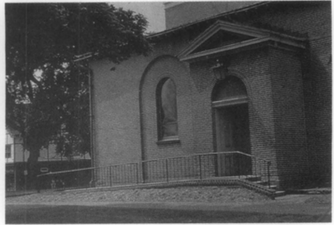
Figure 10. This brick ramp provides access to St. Anne's Episcopal Church in Annapolis, Maryland. Its design is compatible with the historic building. Photo: Charity V. Davidson.
