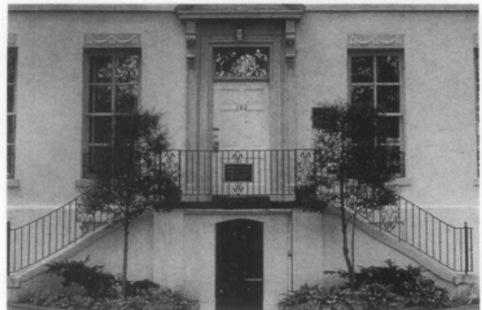
Figure 1. It is important to identify the materials, features, and spaces that should be preserved when planning accessibility modifications. These may include stairs, railings, doors, and door surrounds. Photo: National Park Service files.
