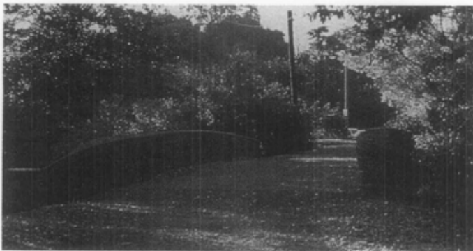
(a.) To improve accessibility in Boston's Emerald Necklace Parks, standard asphalt paving was replaced in selected areas with an imbedded aggregate surface that is more in keeping with the landscape's historic appearance. Photo: Charles Birnbaum.
