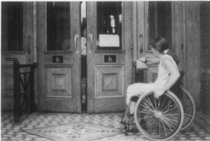
Figure 5. A universal access symbol clearly marks the Arts and Industries Building in Washington, D.C., and a push plate (right) engages the automatic door-opener. Photo: Thomas Jester.
