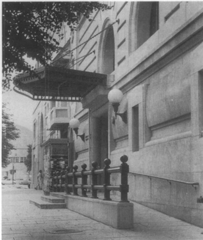
Figure 9. This ramp was created by infilling the window-well and slightly modifying the historic railing. The ramp preserves this building's historic character. Photo: Thomas Jester.
