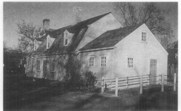
Figure 7. This ramp is convenient for visitors with disabilities and preserves the building's historic character. The design is also compatible in scale with the building. Photo: William Smith.
