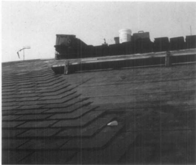
(h) This installation pattern allows the slates to be laid in courses leaving a temporary path of travel to avoid stepping on installed slates.
