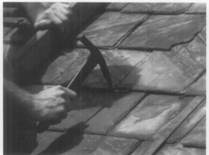
(f) The slate hammer is used to push the bib in place over the nail head.
