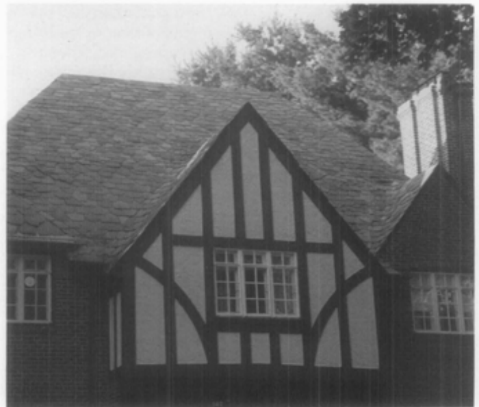
Figure 2. The quaint character of this Tudor style residence is derived, in part, from its textural roof.
