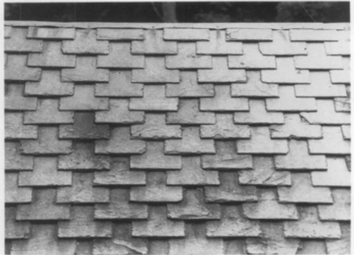
Figure 4. Widely spaced open slating was often used on utilitarian structures where ventilation was desirable. It provided an interesting texture and visual pattern to often plain structures.
