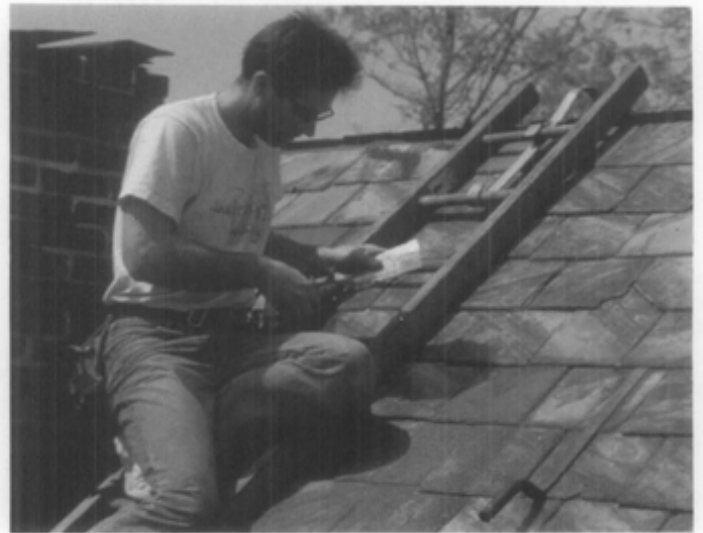
(d) A copper bib is formed to protect the newly created nail hole.
