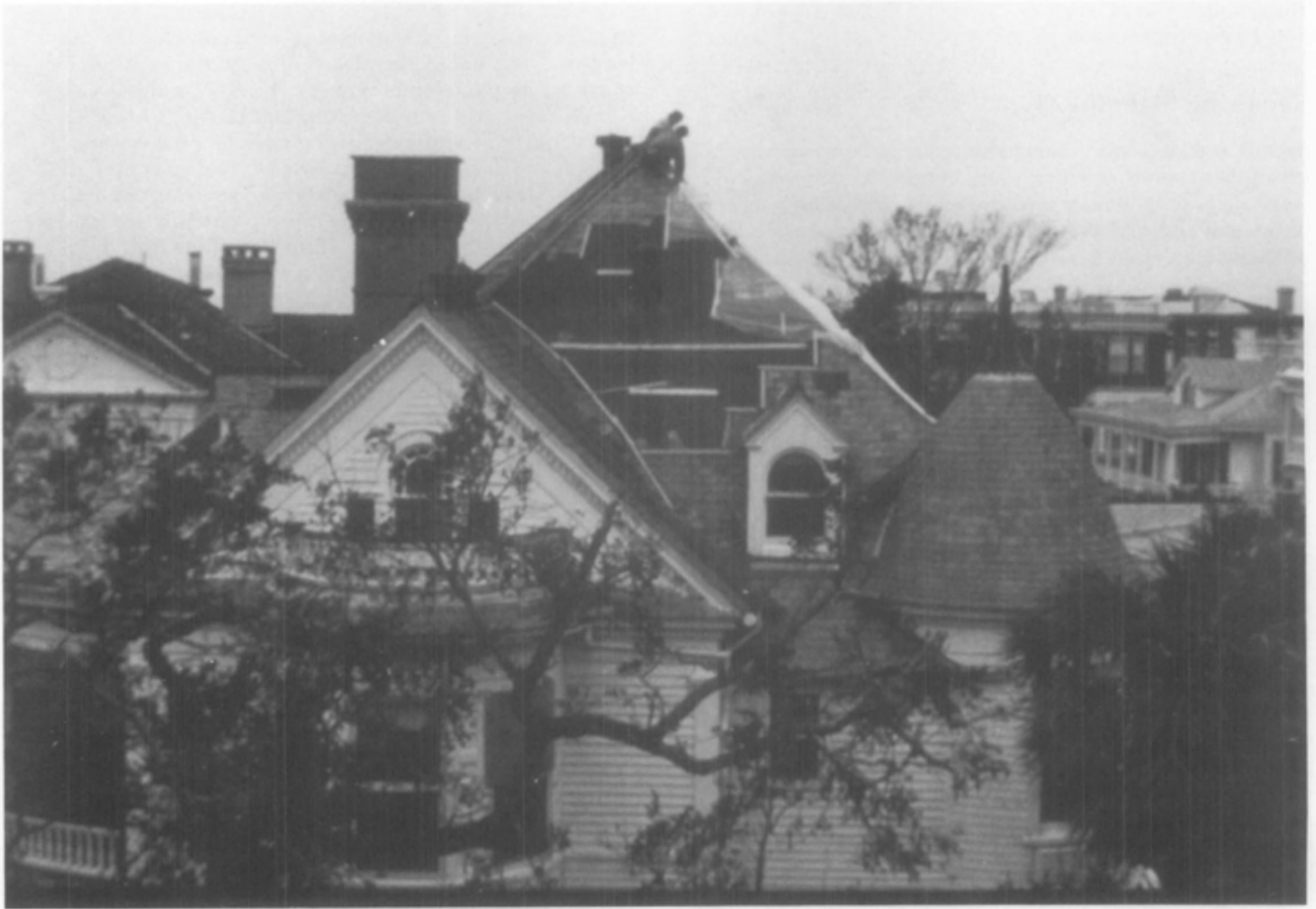
Figure 21. As a result of hurricanes and other disasters, it may be necessary to temporarily stabilize a roof until materials can be obtained and a qualified roofing contractor hired. Heavy roofing felt was stitched into this slate roof to stop moisture penetration until matching slate was obtained for repair. Significant slate roofs should not be stripped off and replaced with asphalt shingles. Photograph courtesy of the National Park Service.
