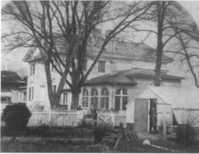
(a) Historic documentation was necessary to determine the historic configuration.
