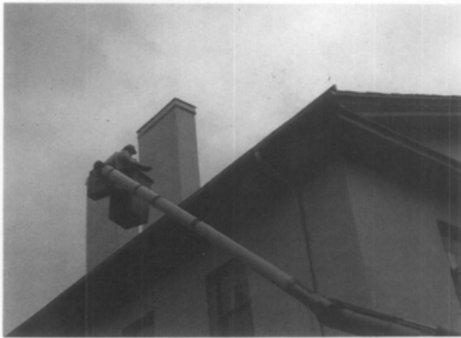
Figure 23. Slate roofs should not be walked on if at all possible. For large projects, lifts can be used to inspect roofs periodically to assess maintenance needs. Photograph courtesy of the National Park Service.
