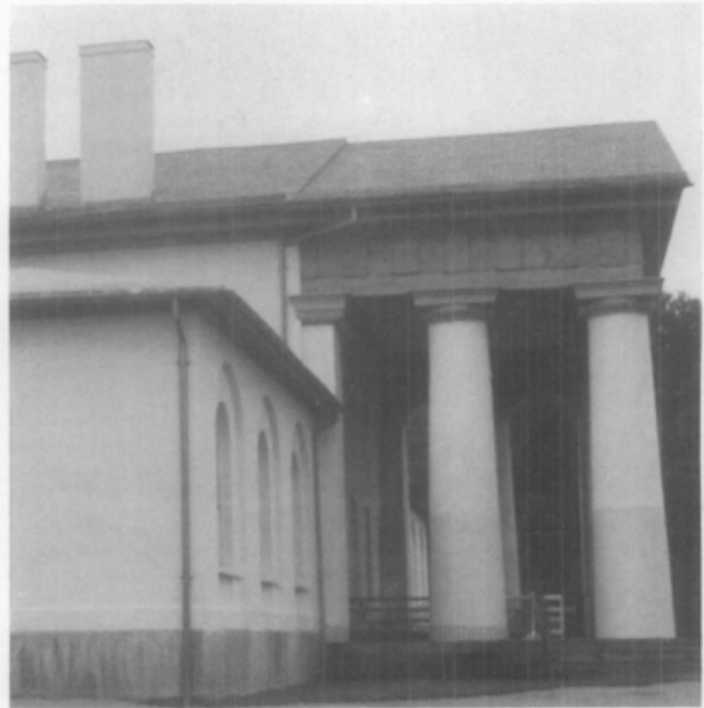
Figure 24. Although slate replacement roofs are expensive, the superiority of materials and craftsmanship will give years of continued service. If amortized over the life of the roof, the replacement cost can be very reasonable. Photograph courtesy of the National Park Service.
