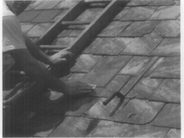
(b) A replacement slate is slid into place.
