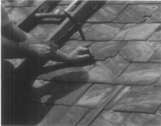
(c) A new slate is secured in place with a copper nail.
