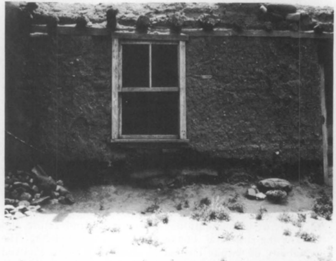
Coving. Salts deposited by rising ground water can evaporate and cause spalling of the adobe bricks at the base of the wall, a serious condition called "coving." Coving can also be caused and/or exacerbated by the erosion of rain splash. (National Park Service)
