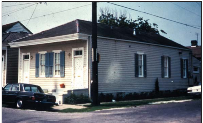
Circa 1900 double shotgun cottage prior to rehabilitation.
