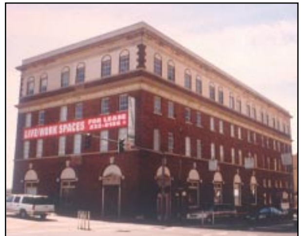
A fourth floor was added in 1934 to this building originally constructed in 1927.
