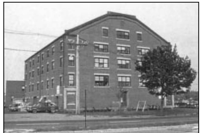
Top: The historically important 1859 brick warehouse with largely solid end wall.
