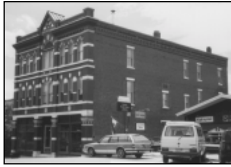
Left: 1882 corner commercial building.
