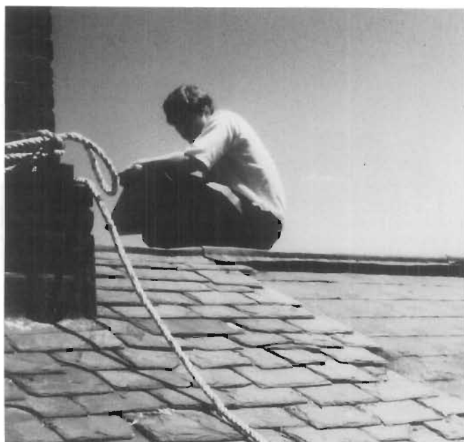
c. Original tinplate roof beneath slate (John G. Waite)
