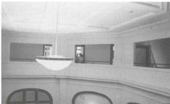
Second floor openings in the atrium were restored to their original size, and a simple railing added to the sill to meet code requirements.
