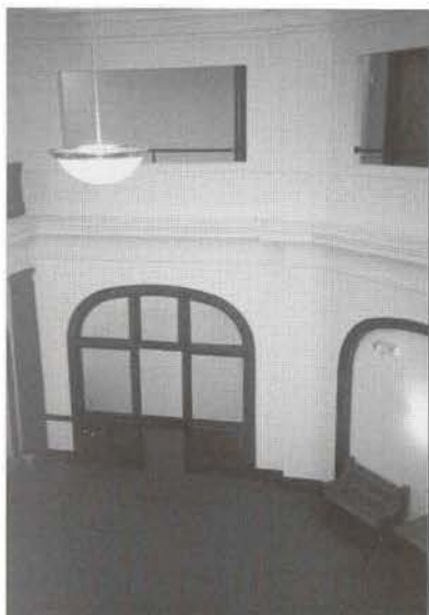
The atrium space after rehabilitation
