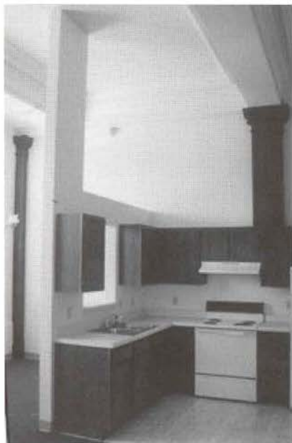
The historic beamed ceilings and trim remain visible by constructing low dividing walls approximately six feet below original ceiling heights, and by not lowering the ceilings in primary spaces.
