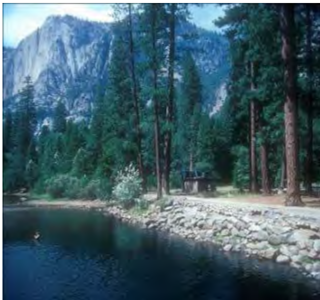
Figure 1: Riprap and paved path on bank below Housekeeping Bridge prior to restoration.
