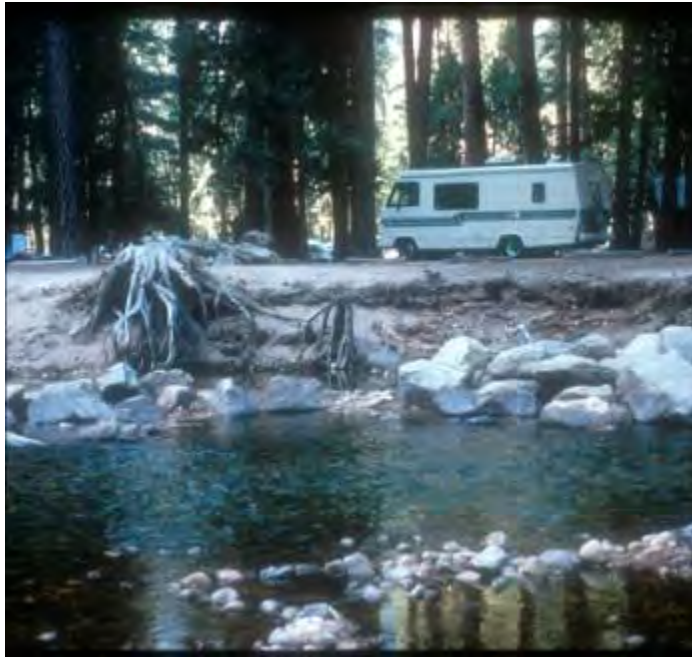
Figure 1: Riverbank at Lower River Campground before restoration, 1991. Note the displaced riprap in the river channel.
