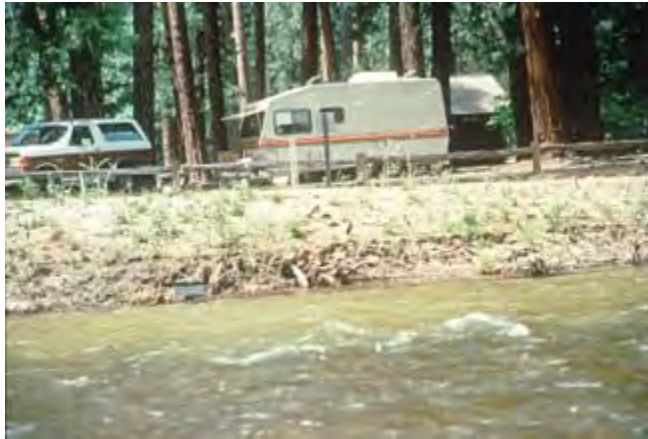
Figure 3: Lower River Campground 1 year after restoration.
