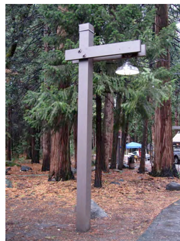
Figure 1 Rusticity: wood post structure, Hetch Hetchy, with an industrial style luminaire
